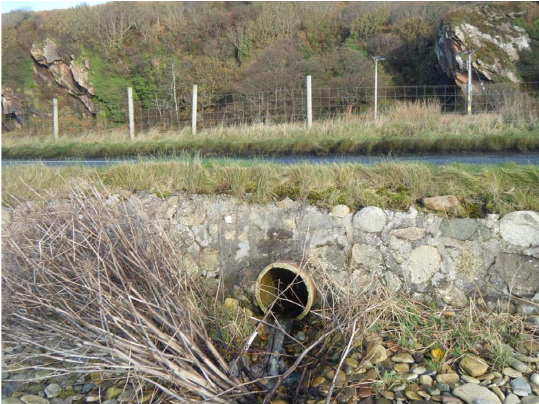
Figure 22. 32cm diameter pipe
