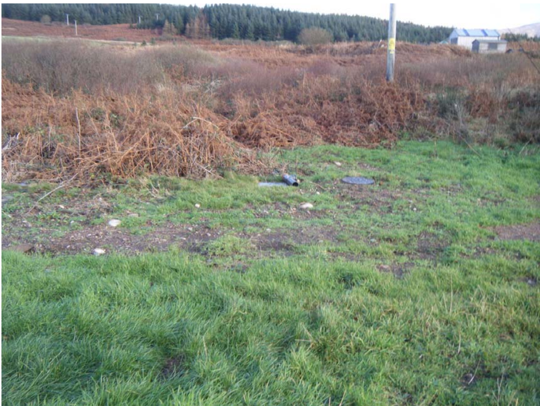
Figure 17. Septic tank for golf course clubhouse
