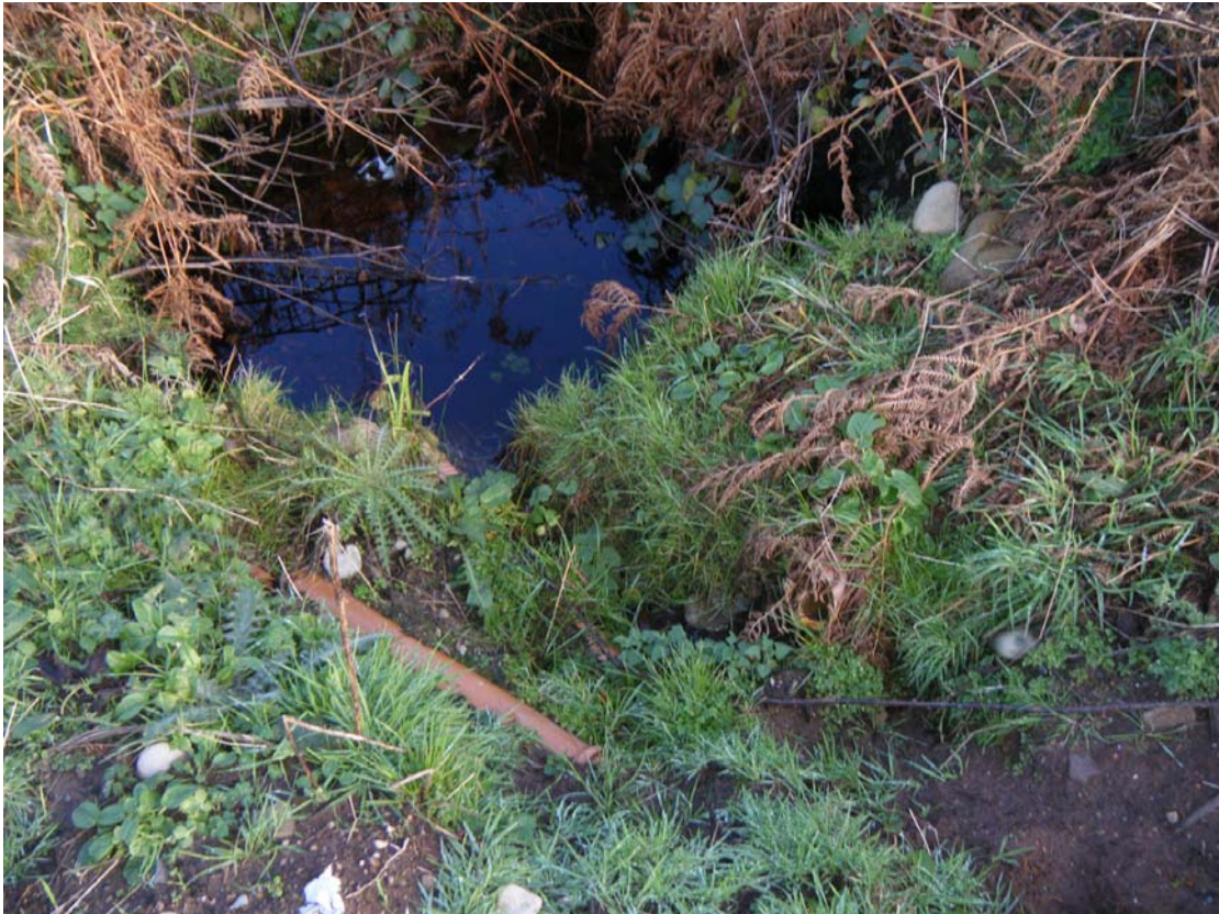
Figure 18. Septic tank outfall for clubhouse leading into small stream
