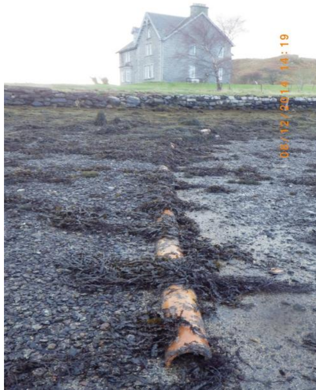
Fig 8. House at Mount Pleasant with pipe onto shore, no flow was observed, associated with waypoint 20.
