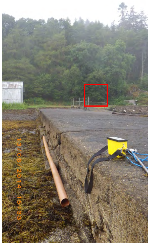
Figure 8: PVC discharge pipe on side of pier, with fibre glass tank present on upper shoreline (centre right within red box). WP 22
