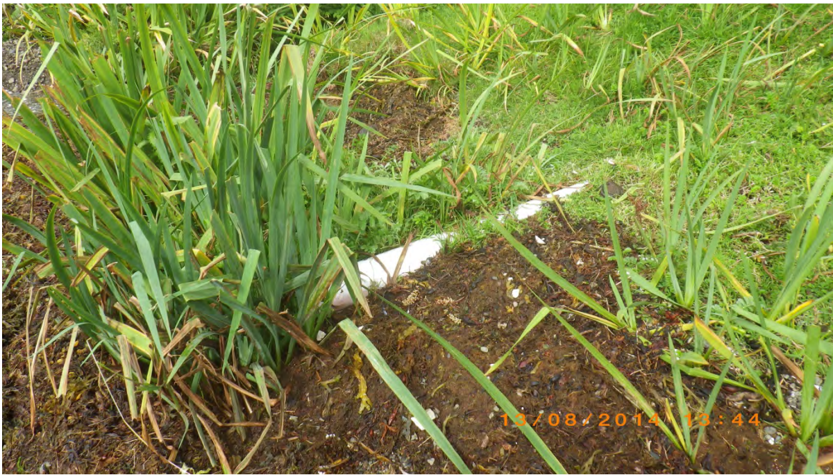
Figure 5: PVC pipe running to shoreline below house on shoreline. End obscured by reeds, but no discharge. WP 7
