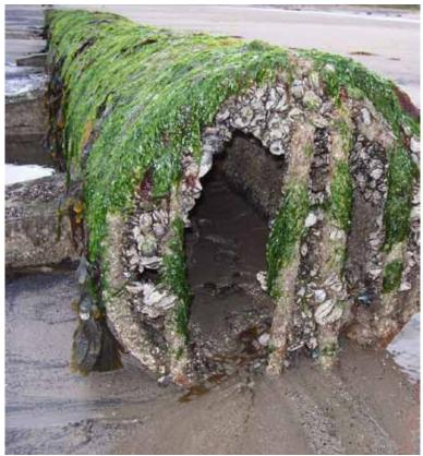
Figure 6. Outfall pipe with mussels growing around the edge
