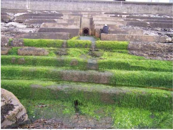
Figure 15. Outfall pipe with evidence of faecal contamination
