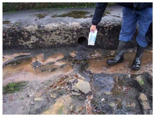
Figure 18. Outfall pipe with slight flow
