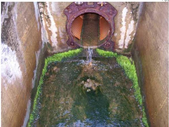
Figure 16. Evidence of faecal contamination in top outfall shown in Figure 15
