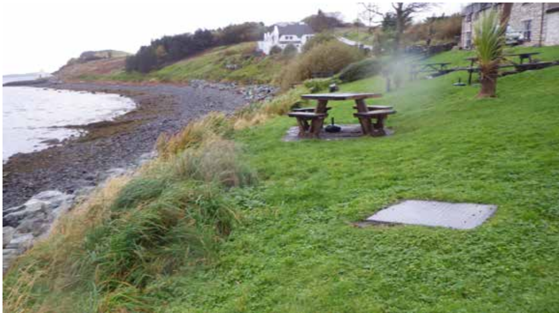
Figure 14. Manhole cover above shore, below Stein Inn. No discharges onto shore below. Associated with waypoint 32.
