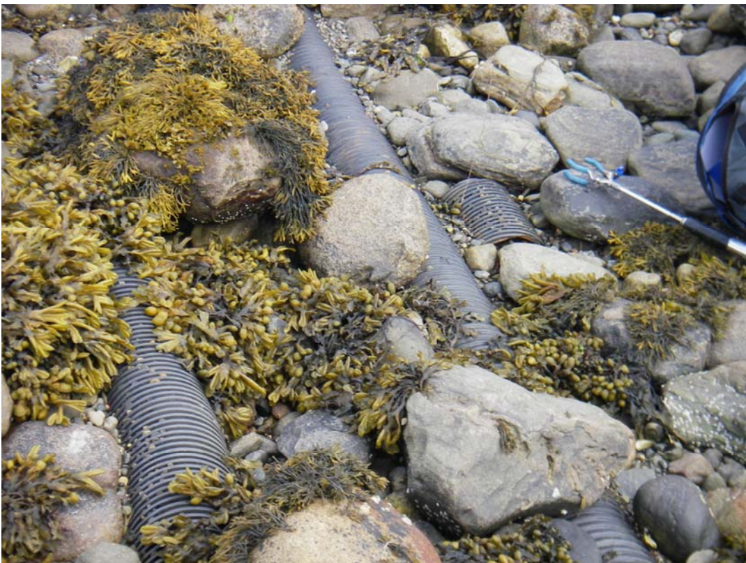
Figure 13. Possible septic discharge pipe
