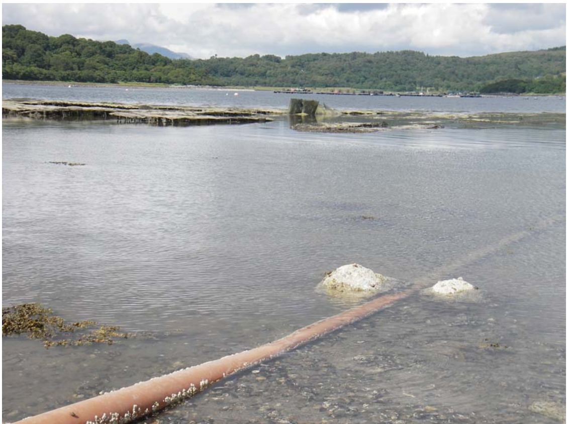
Figure 23. Presumed sewer pipe at Shian Fisheries
