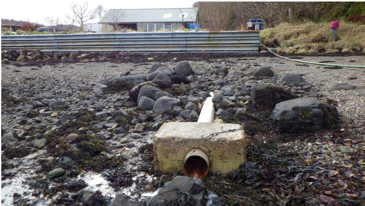
Figure 18. Second large outflow from processing farm. Waypoint 23.
