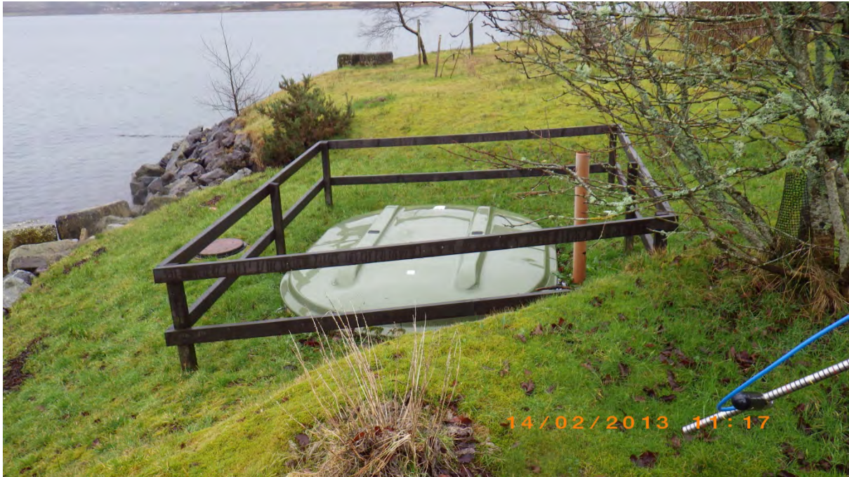
Figure 31. Septic tank outside Scottish Sea Farms. Waypoint 98.
