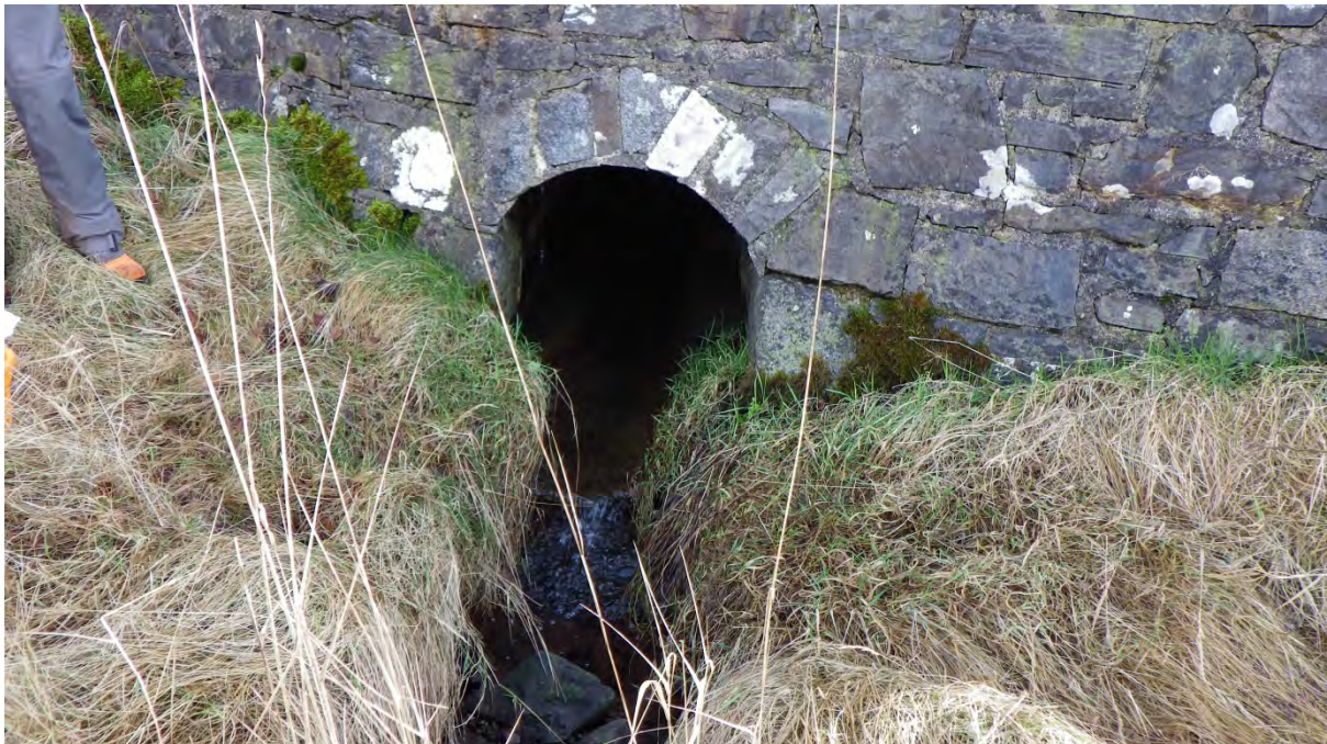
Figure 14. Small burn runs into bay through culvert. Waypoint 16.
