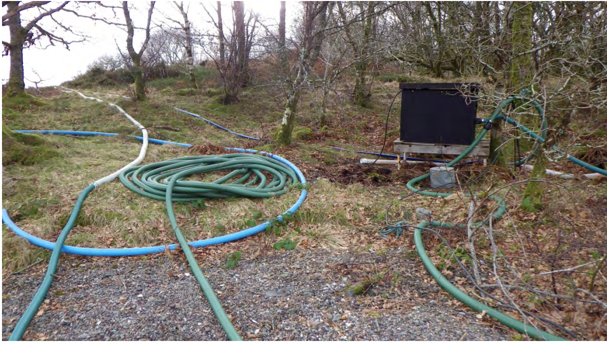
Figure19. Pipework running to and from processing yard. Waypoint 23.
