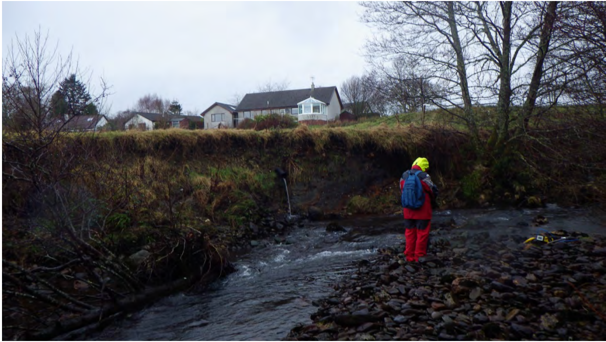
Figure 27. Plastic corrugated pipe possibly land drain with smell. Waypoint 74A.
