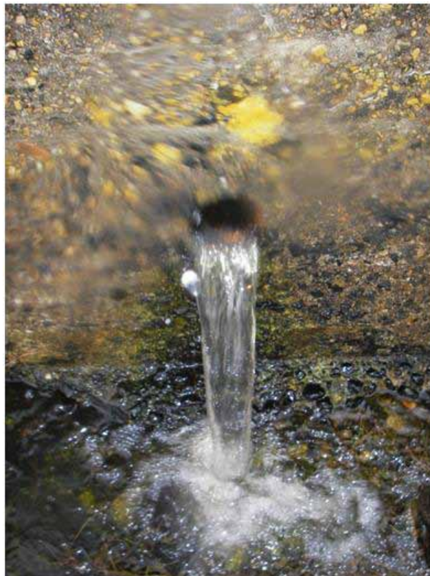
Figure 13. Piped flow from sea wall
