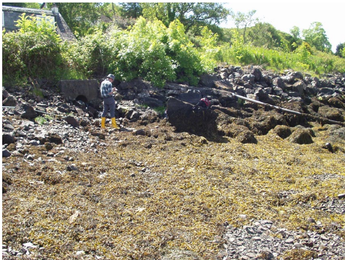
Figure 6. 60cm culvert and plastic pipe leading down to sea, end submerged
