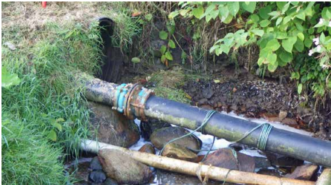
Figure 16. Watercourse running from side of Loch Fyne Oysters. Associated with waypoint 87. Location of sample LFFW7.
