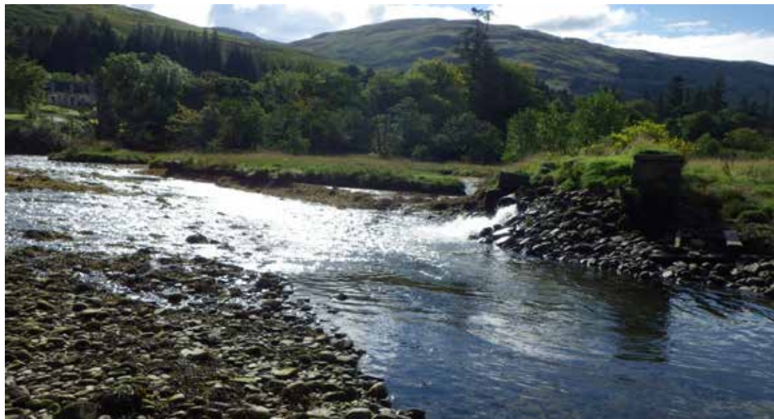
Fig 8. Watercourse diversion through large plastic pipe. Associated with waypoint 31. Location of sample LFFW3.
