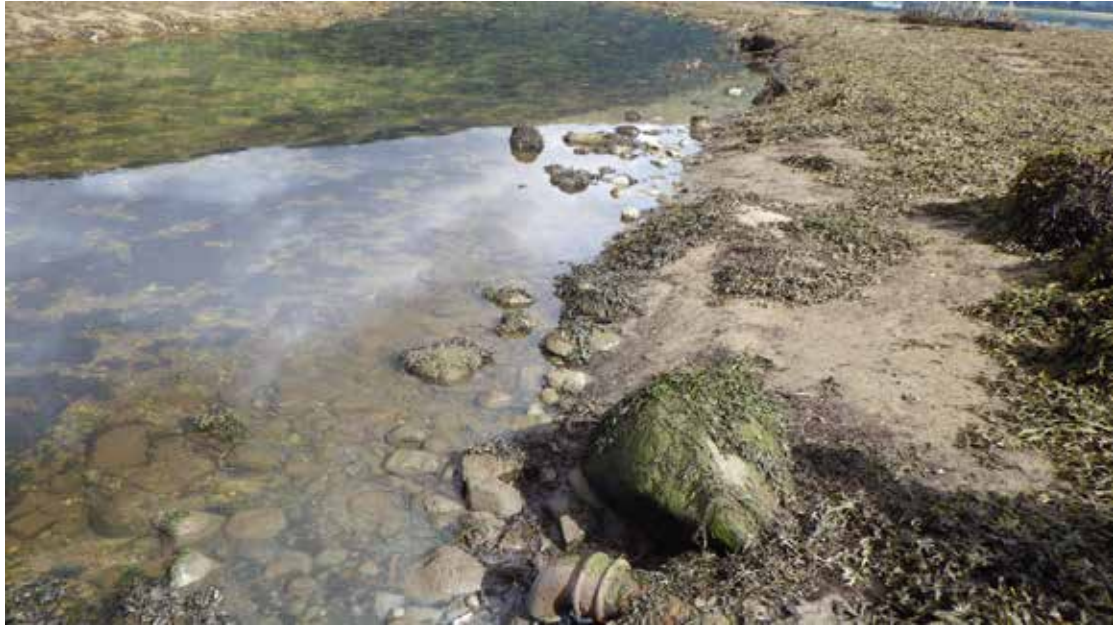
Figure 9. Clay outfall pipe into river. Associated with waypoint 40. Location of sample LFFW4.
