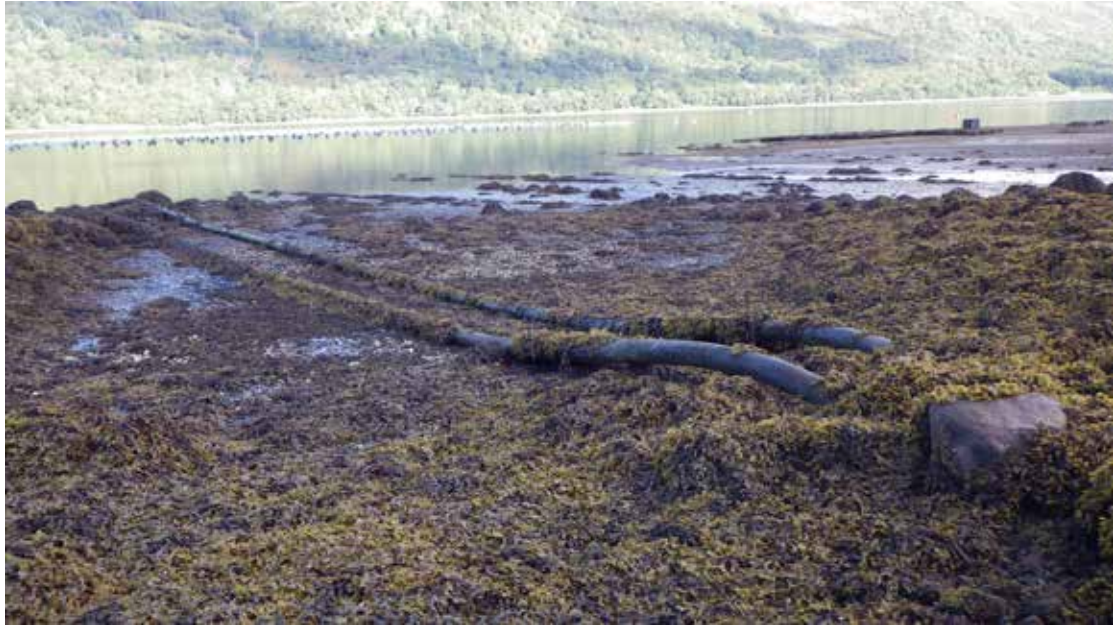
Figure 15. Inlet and outlet pipes from Loch Fyne Oysters. Associated with waypoint 85.
