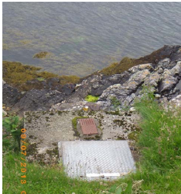
Figure 5. Manhole cover with pipe. Waypoint 16.
