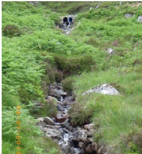
Figure 12. Two pipes under service road above sample site LGFW7. Waypoint 42.
