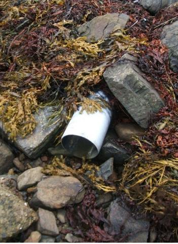
Figure 17. Probable septic tank outlet
