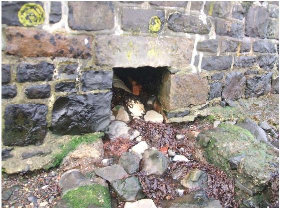
Figure 11. Probable septic tank outlet
