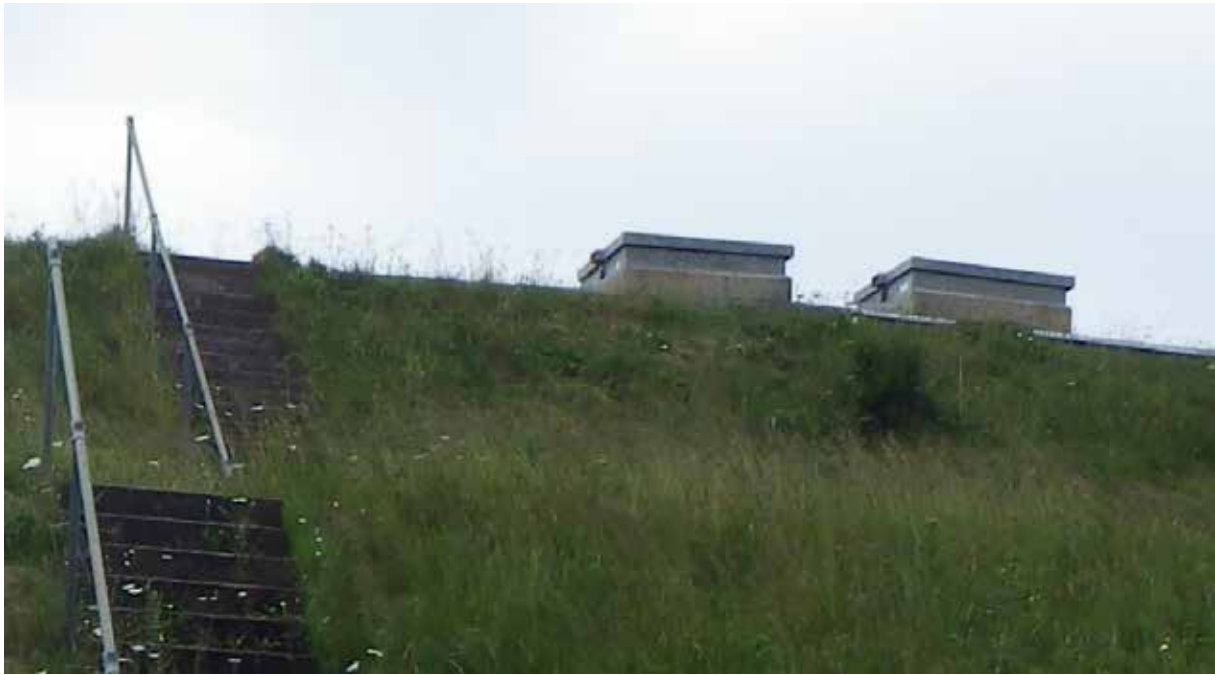
Figure 12. Septic tanks. Waypoint 42.
