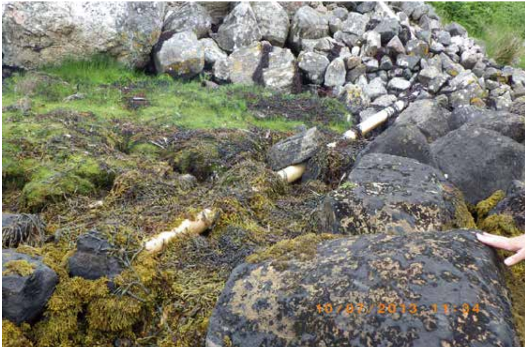
Figure 18. Pipe running to shore from house, Unplanned Seawater Sample LI2SW1. Waypoint 70 & 71.
