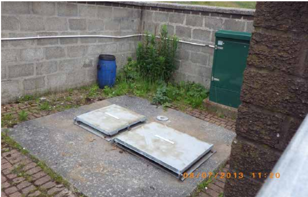
Figure 8. Septic tank storage area. Waypoint 32.
