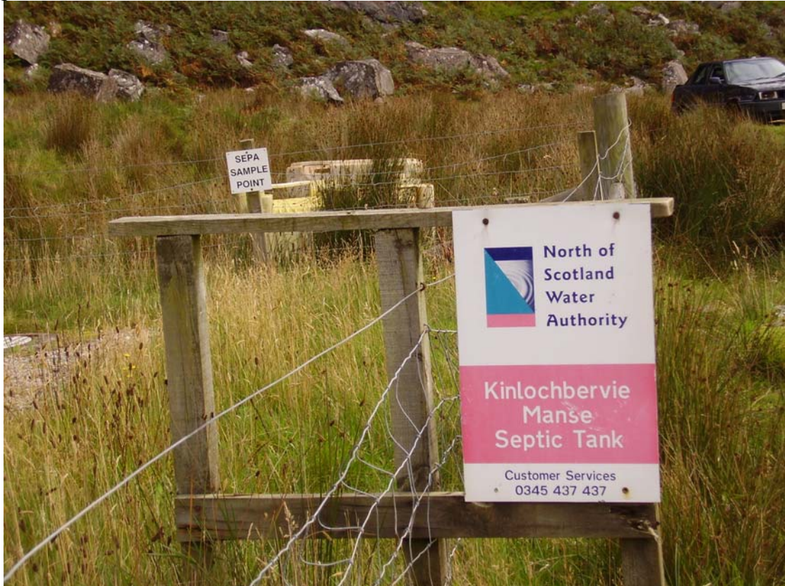
Figure 26. Kinlochbervie Manse septic tank.
