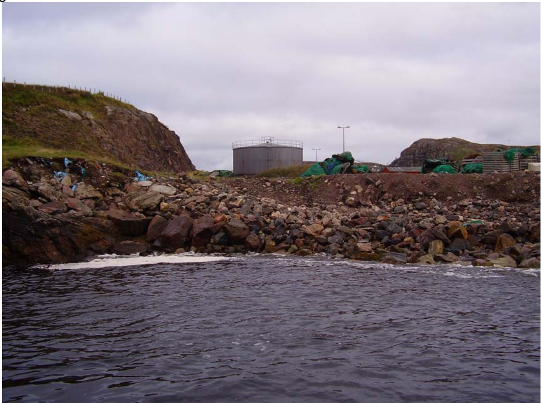
Figure 16. Kinlochbervie ST outfall near here.
