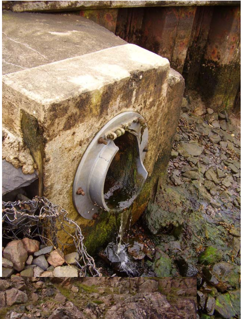
Figure 22. Discharge from near corner of pier.
