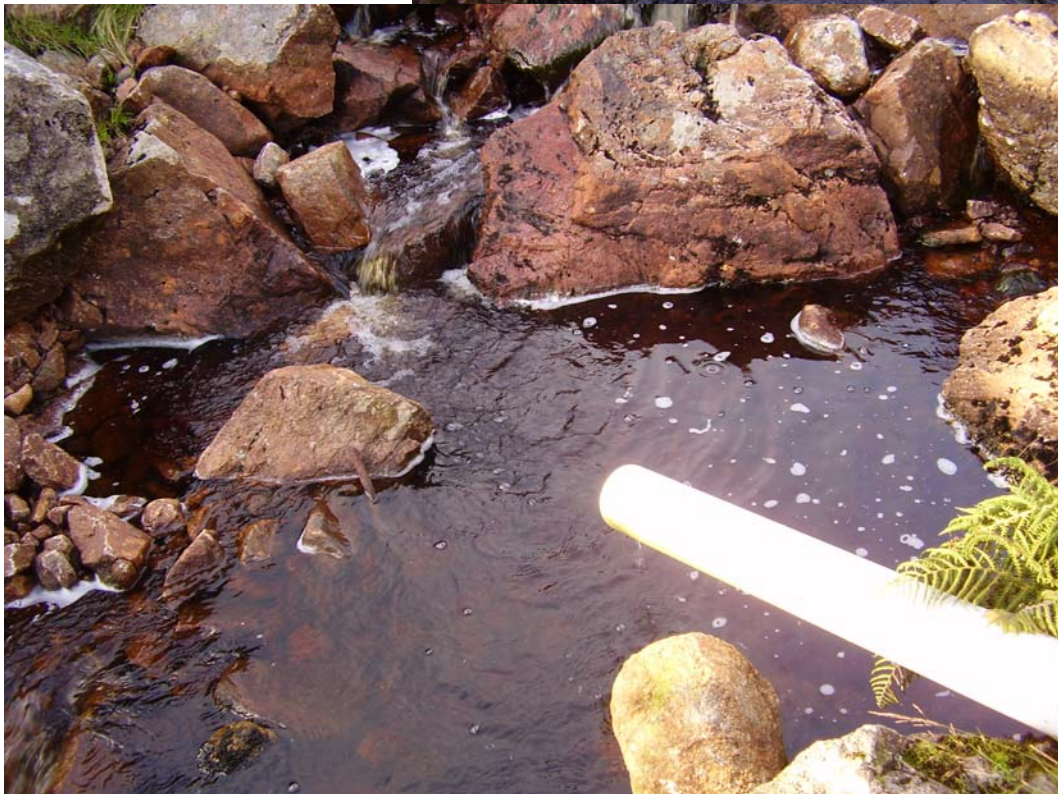
Figure 35. Septic pipe discharge
