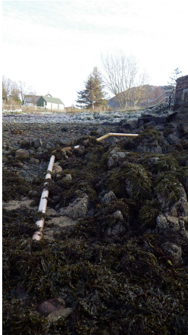
Figure 11: Plastic outflow pipe not on original map with no obvious discharge (Waypoint 15)
