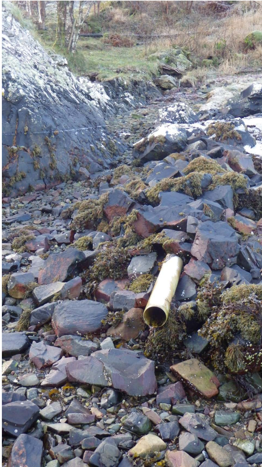
Figure 7: Plastic pipe discharging on to shore (Waypoint 5)
