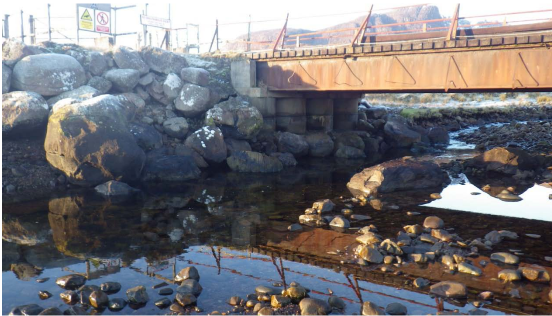
Figure 14: Road bridge leading to restricted site with river running beneath (Waypoint 25)
