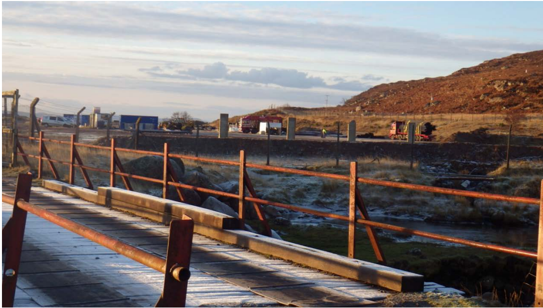
Figure 16: Road bridge leading to restricted site (Waypoint 25)
