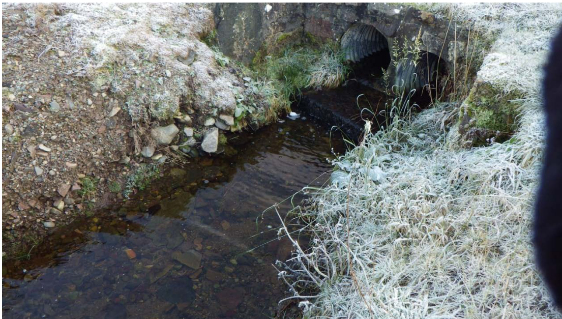
Figure 9: Culvert running under road (Waypoint 8)
