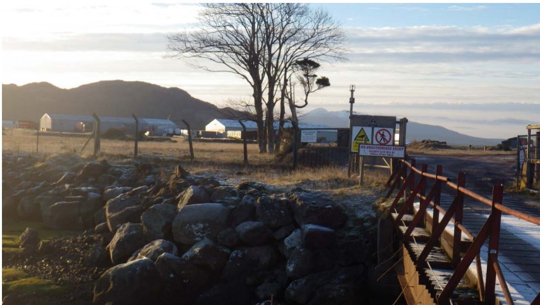
Figure 15: Road bridge leading to restricted site (Waypoint 25)
