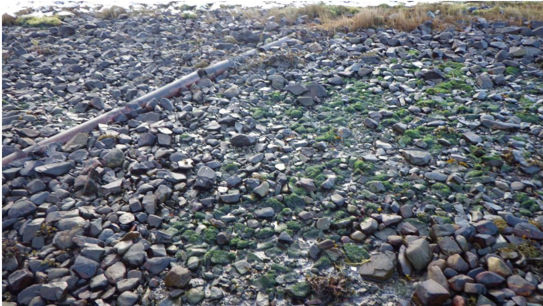
Figure 8: Broken clay pipe and green algae ( Ulva sp.) on shore (Waypoint 6)
