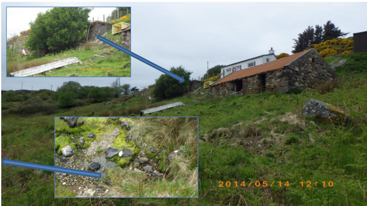
Fig 23. Foindle septic tank and apparent soak away at NC 1925 4881. Bottom blue arrow shows seepage onto shore at Waypoint 98.
