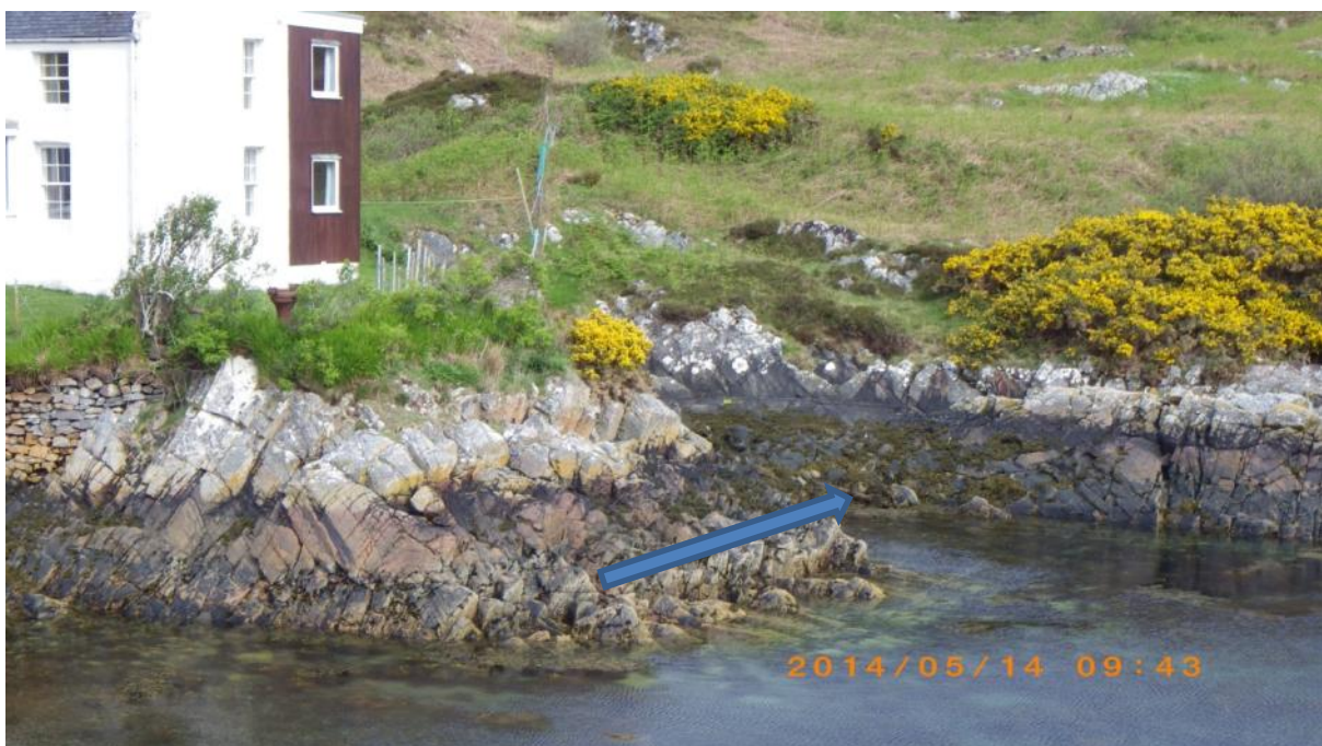
Fig 19. Blue arrow indicates outflow pipe from property above the shore associated with waypoint 81 & 82.
