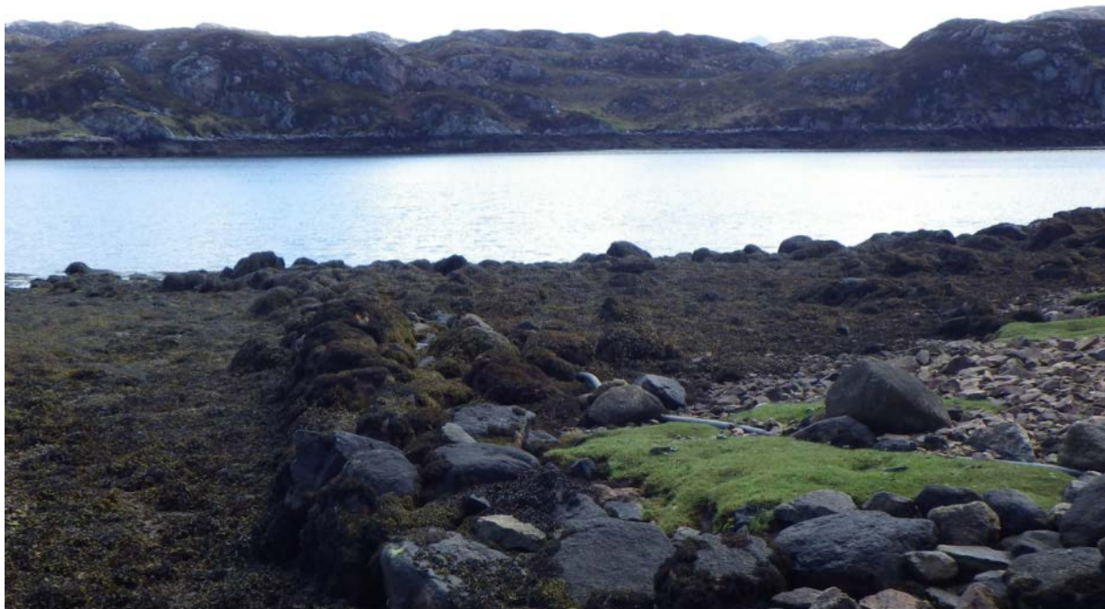
Fig 7. Permitted private shore outfall in 50 mm alkathene pipe. Associated with Waypoint 4.
