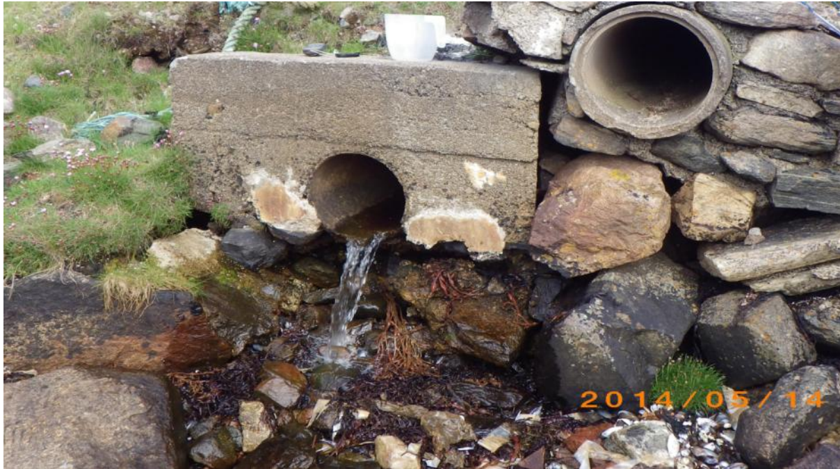
Fig 18. Concrete pipe road culvert with flow. Location of sample LLFW2, Waypoint 81 & 82.
