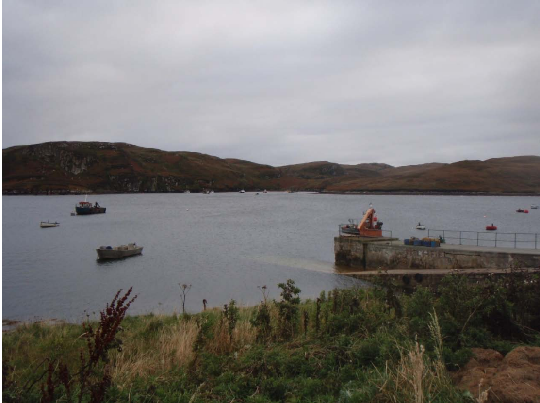
Figure 18. Crosbost jetty, view of boats moored on opposite side of loch
