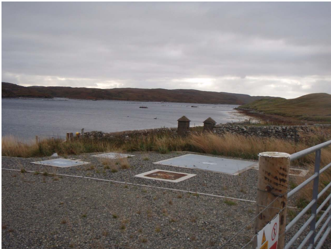
Figure 16. Septic tank with mussel farms visible in background
