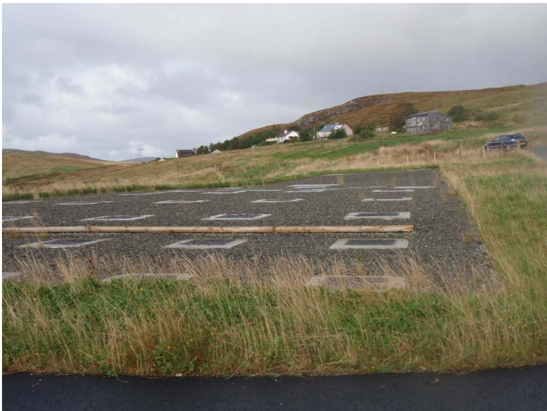
Figure 12. View looking north across septic tank installation toward road
