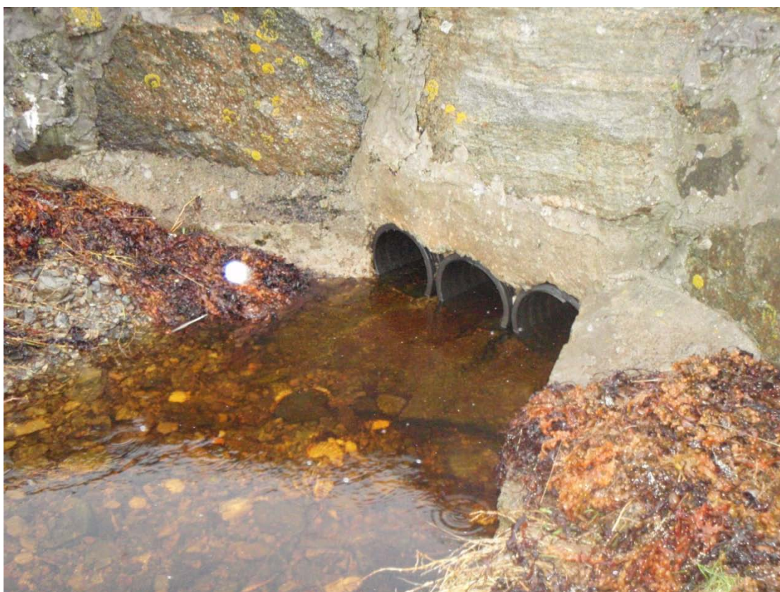
Figure 17. Stream flowing through culvert, East Crosbost
