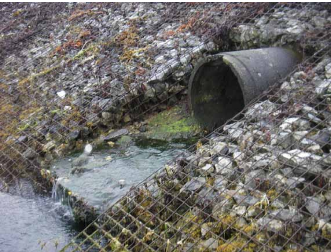
Figure 8. Stream running through concrete pipe
