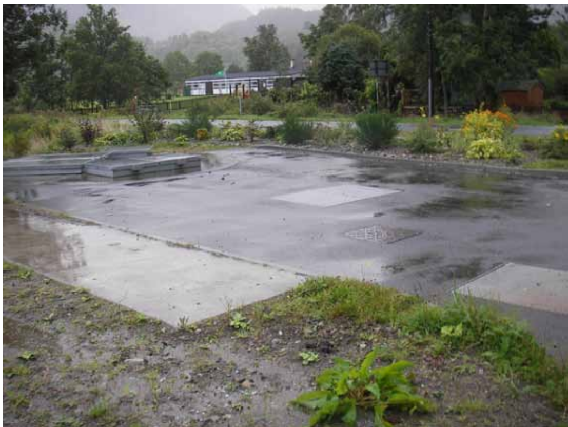
Figure 10. Part of Glencoe Waste Water Pumping Station site
