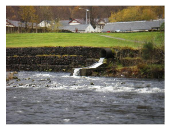
Figure 18 Surface water outfall
