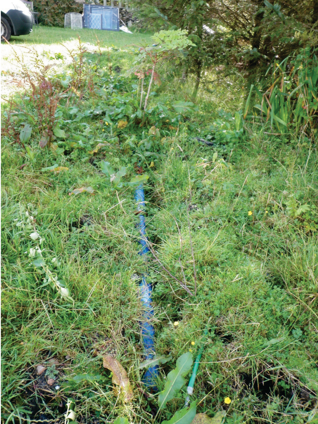
Figure 17. Blue pipe, purpose not known, could not locate end
