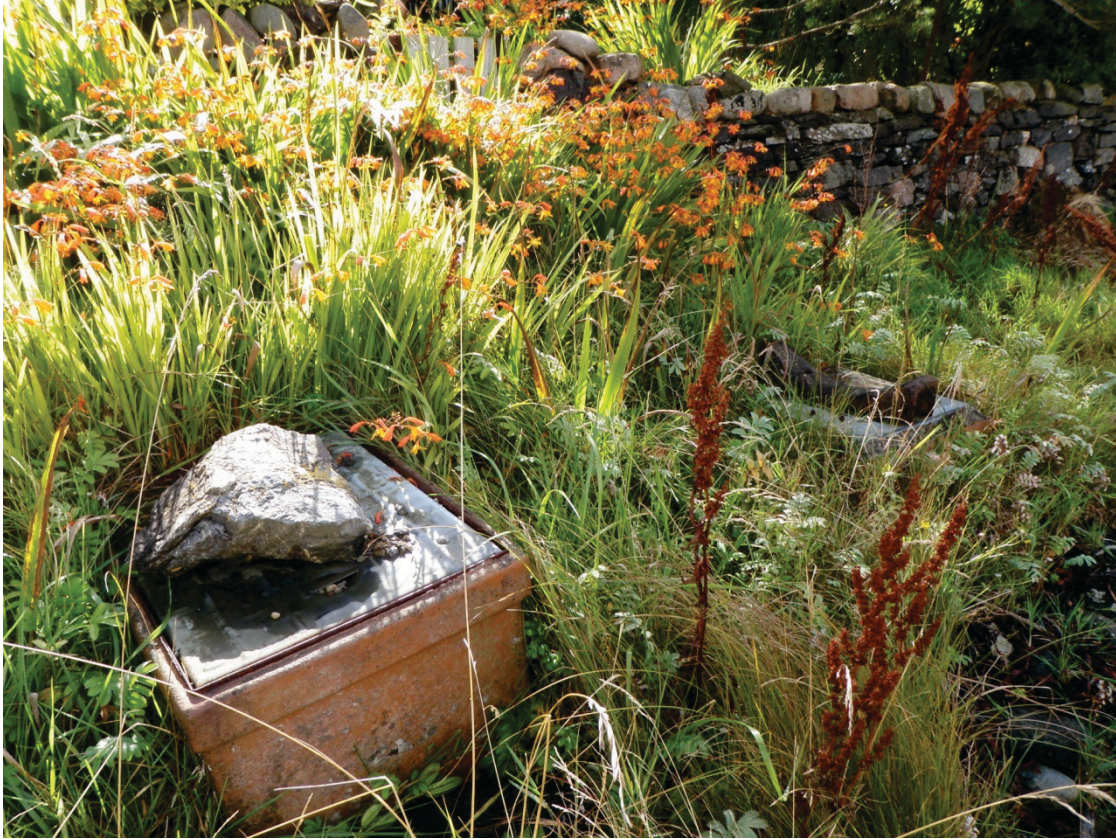
Figure 14. Two septic tanks, no sign of outfall pipes
