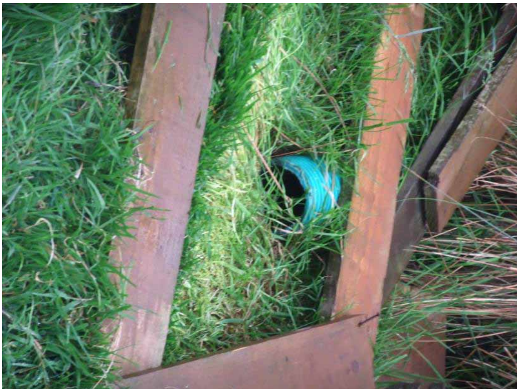
Figure 16. Drainage pipe below septic tank
