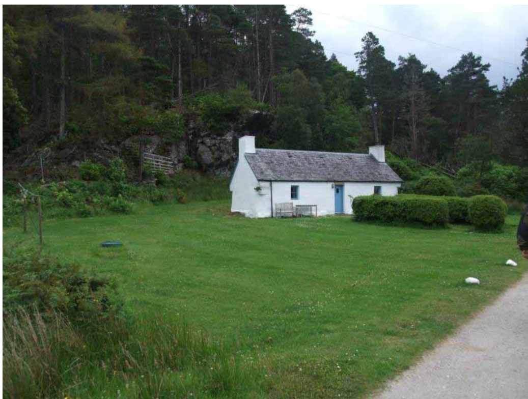
Figure 9. Small cottage with septic tank in garden
