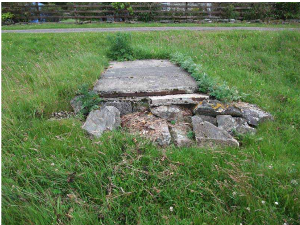
Figure 8. Septic tank near high tide mark
