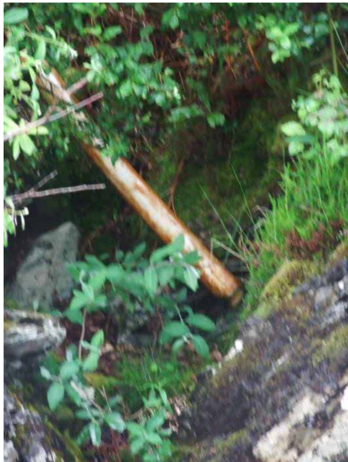
Figure 19. Outfall pipe from septic tank
