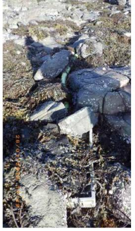
Figure 8: Plastic pipe and intake box on shore at Eilean Casach fish farm (Waypoint 28)
