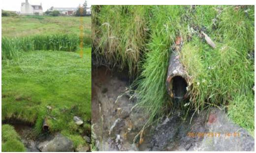
Figure 18. Pipe discharging into watercourse from below house. Waypoint 38.
