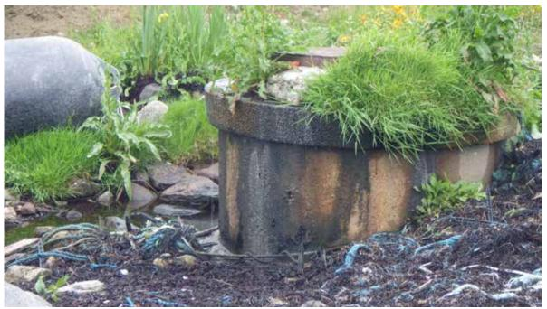
Figure 5. Outfall pipe discharging into watercourse. Waypoint 5.
