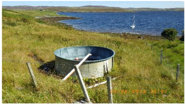
Fig 11: Large, open tank below public road, with pipe and inflow running in.
