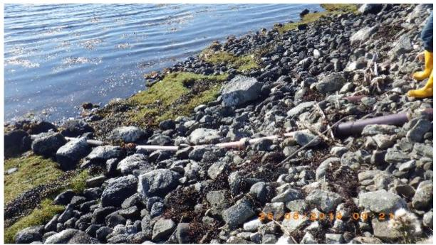
Fig 16: Pipe running from foreshore into bay with end below sea level, WP62. No flow observed at broken section on upper shore.
