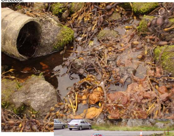
Figure 35. Roag080765 Septic discharge with human waste on shoreline, N of Circebost.
