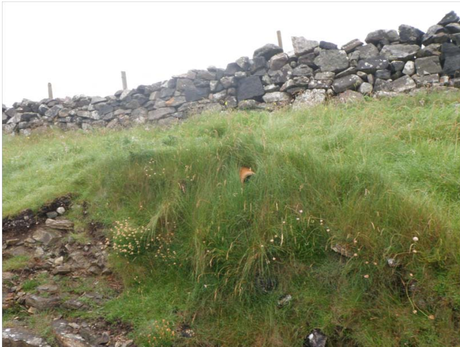
Figure 4. End of ceramic septic pipe
