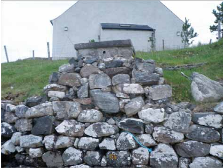
Figure 10. Septic tank with dry overflow above shoreline
