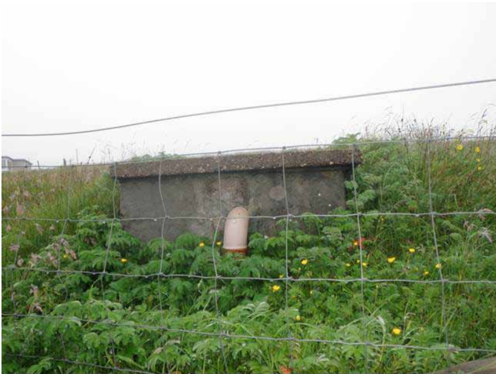
Figure 5. Septic tank above shoreline
