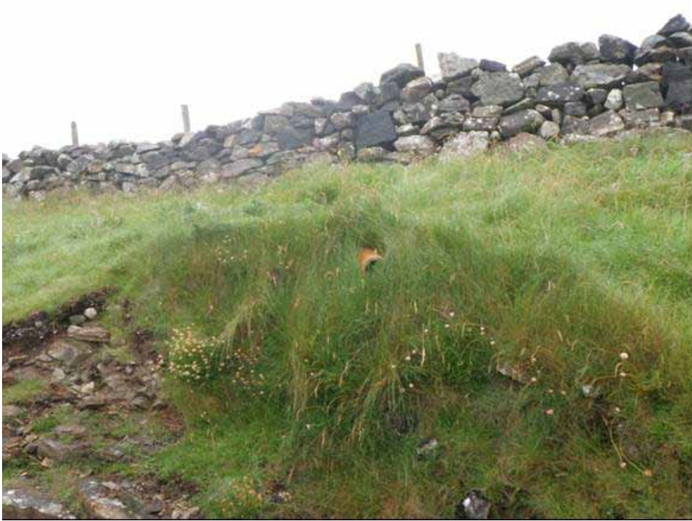
Figure 4. Dry end of discharge pipe
