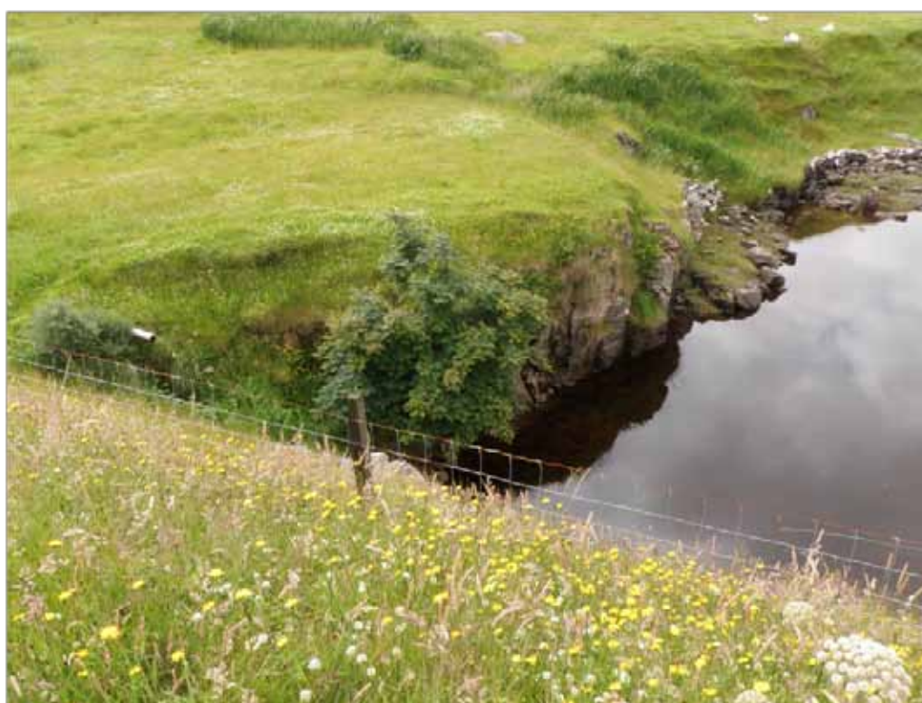
Figure 17. Discharge pipe to ponded end of Abhainn Uasaig
