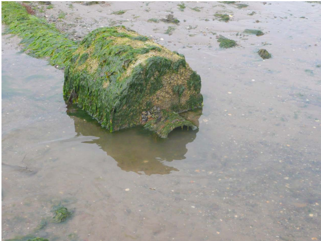
Figure 6. End of outfall pipe
