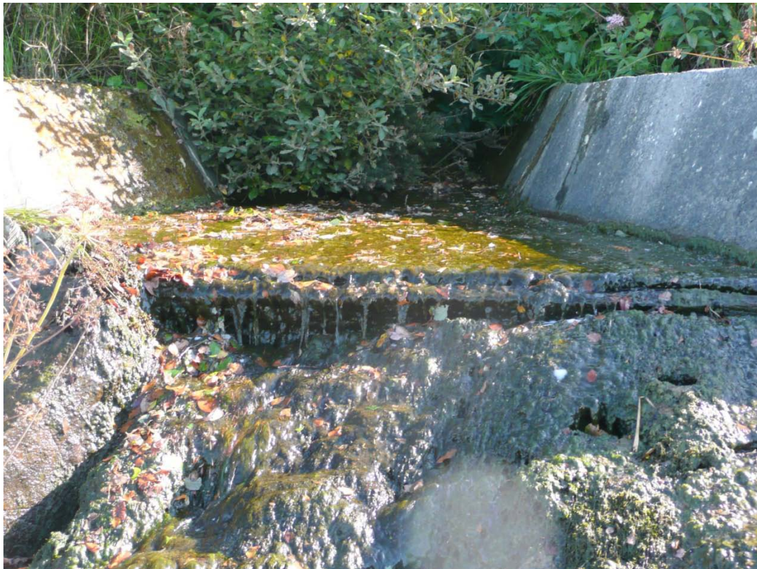
Figure 14. Culvert, location of water sample LR016
