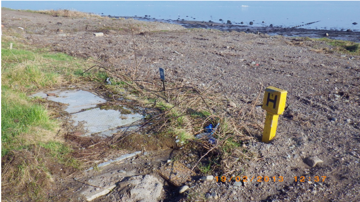
Figure 7. Manhole cover is freshly flattened area along the shore. Waypoint 10.
