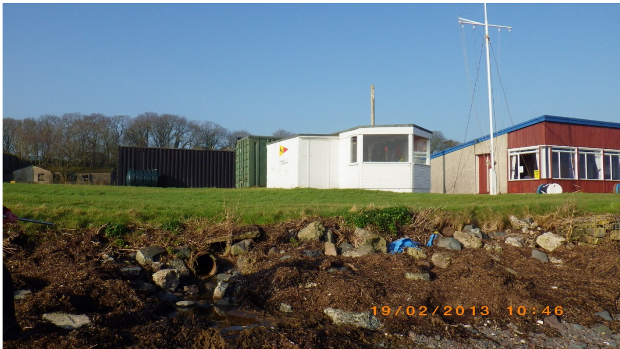
Figure 3. Large clay discharge pipe at Loch Ryan Sailing Club. Waypoint 1.
