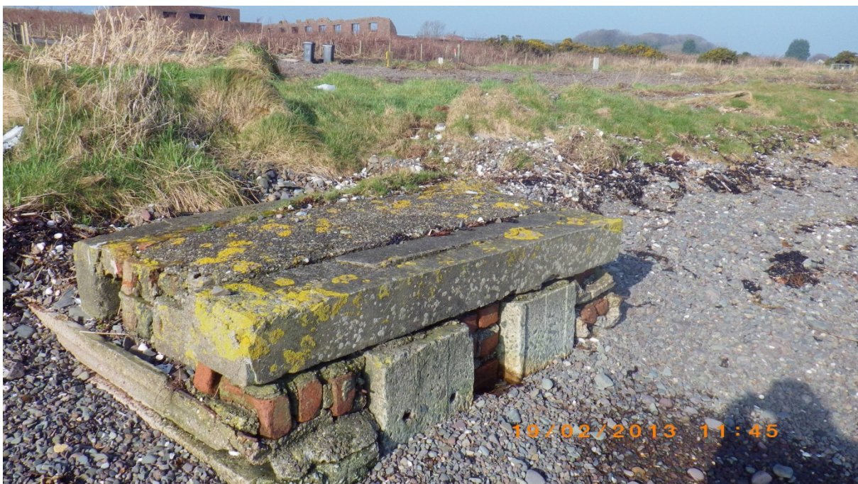
Figure 8. Concrete structure most likely associated with sewage work. Waypoint 11.
