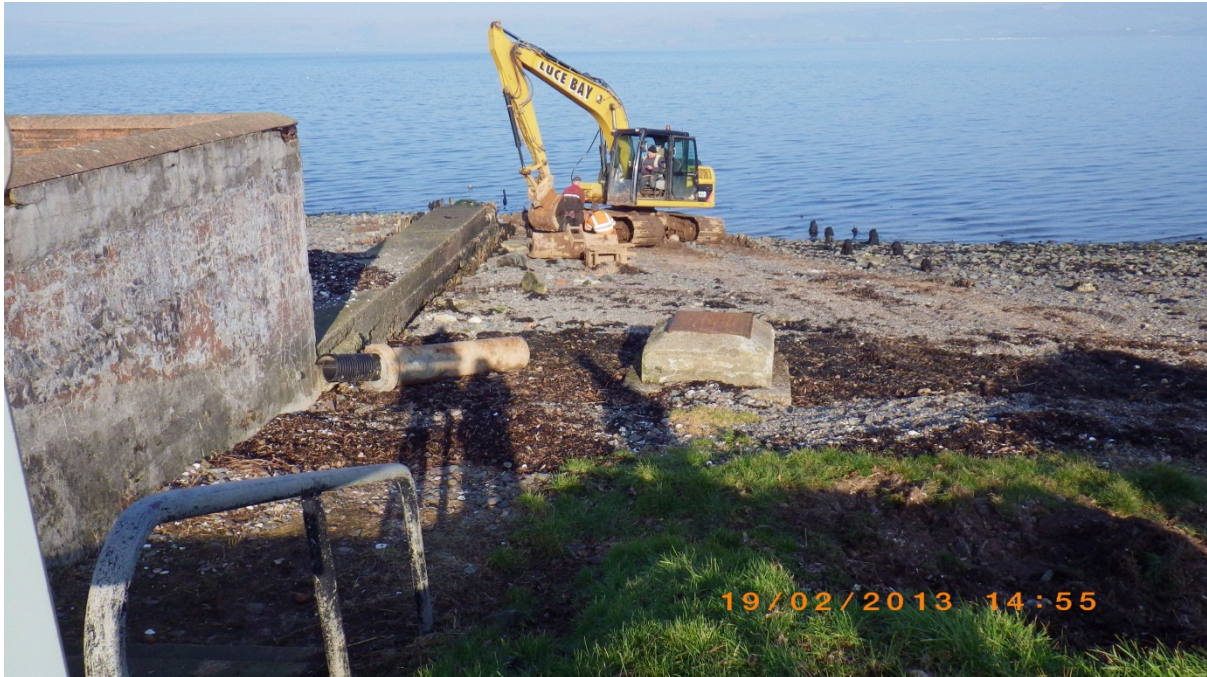
Figure 15. Pipe replacement work. Waypoint 24.
