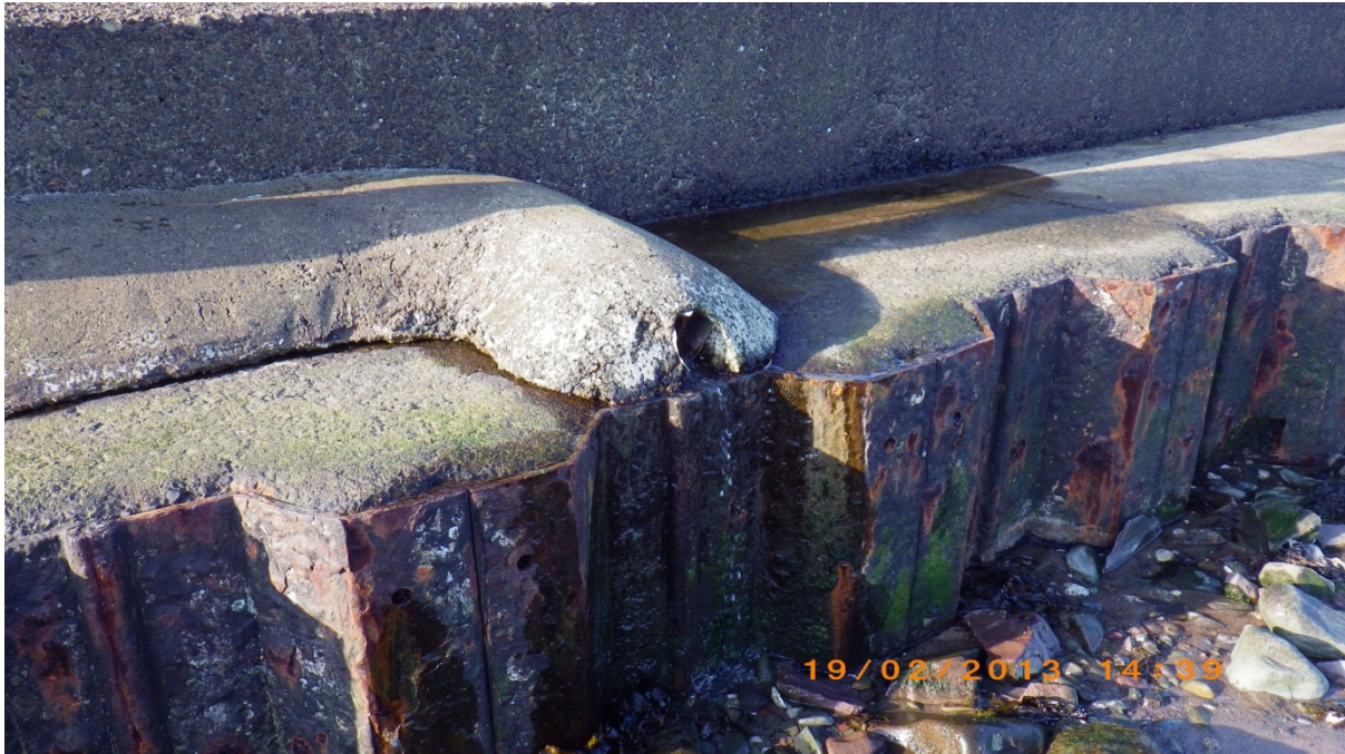
Figure 12. Small pipe with outflow in seawall along the shore in town. Waypoint 21.
