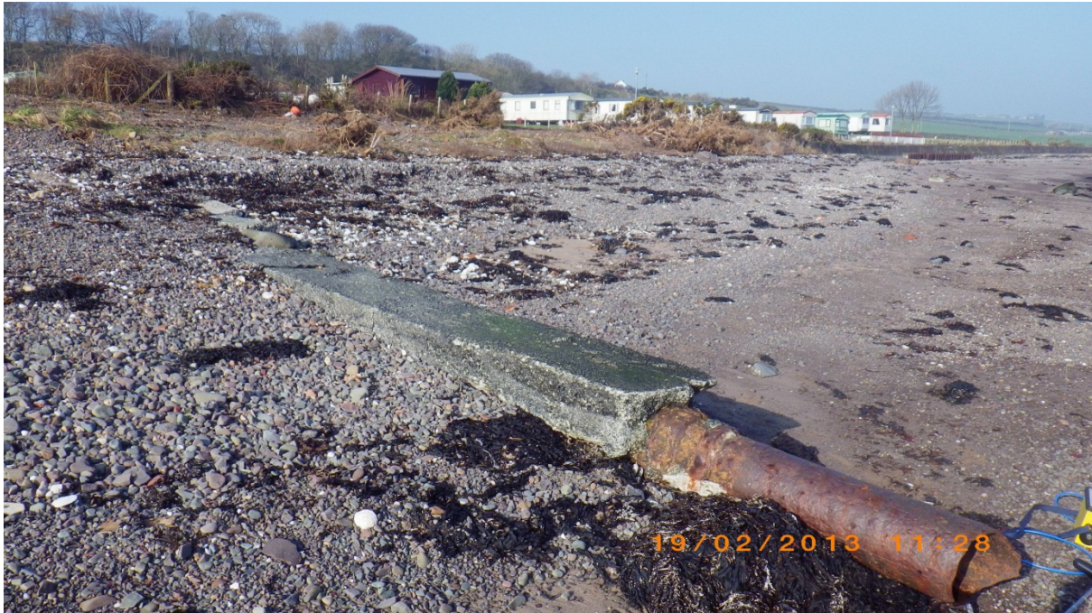
Figure 5. Large metal outflow pipe at the entrance to caravan site. Waypoint 8.
