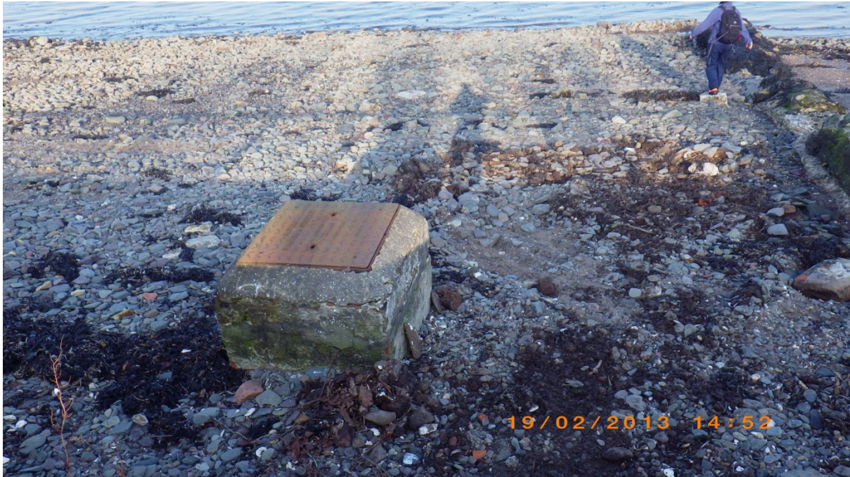
Figure 14. Old metal pipe in concrete with manhole cover. Waypoint 23.
