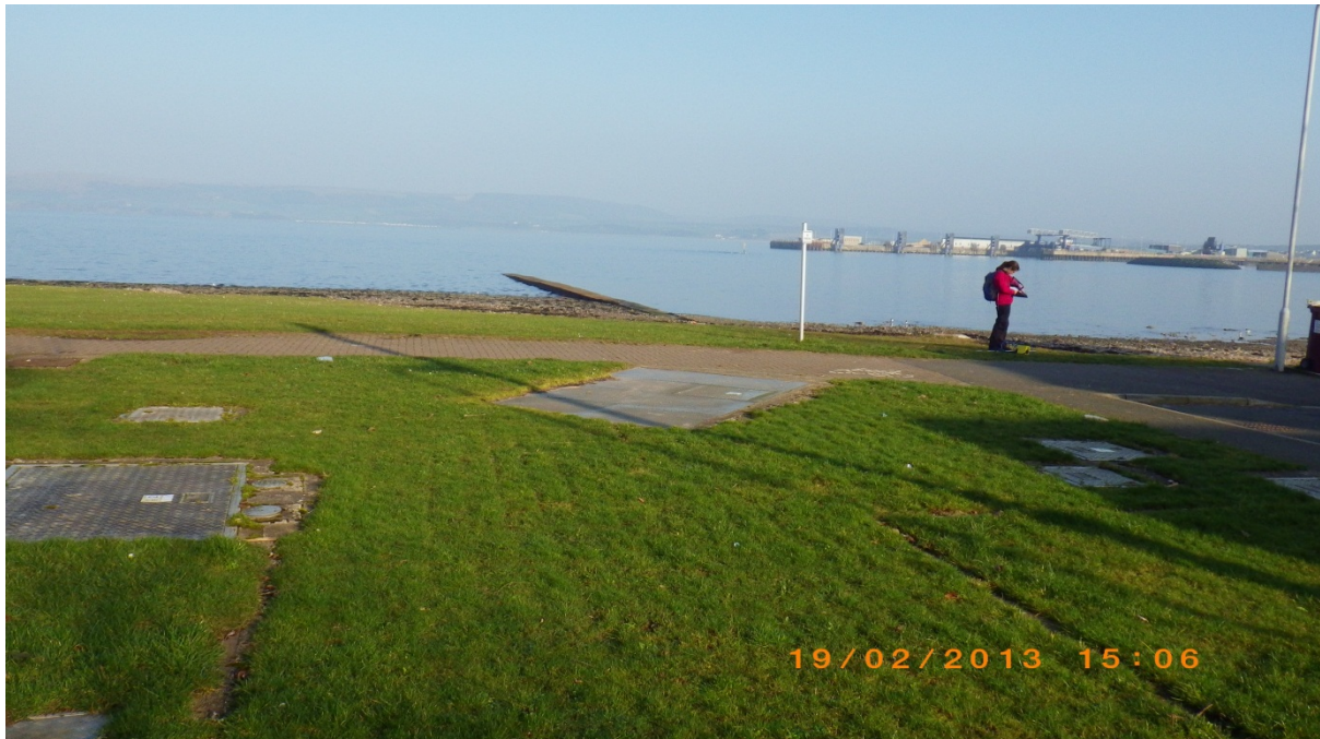
Figure 19. Manhole covers at pumping station. Waypoint 26.
