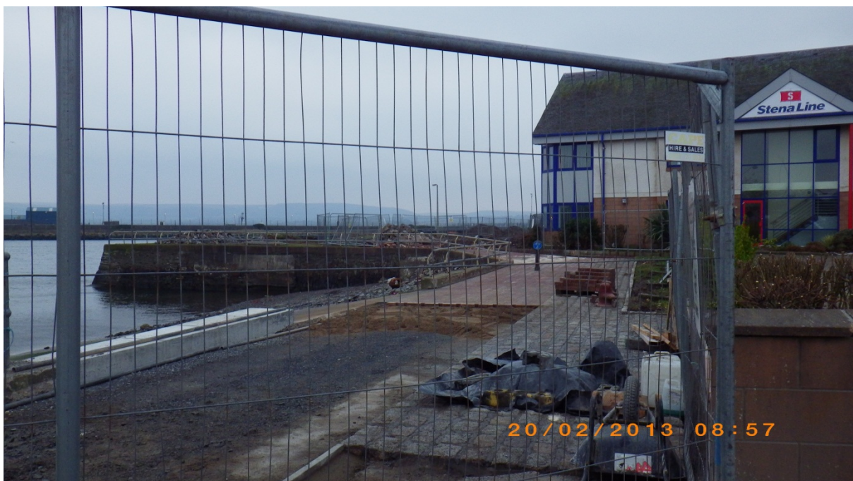
Figure 20. Closed access to shore around Stena Line office in Stranraer. Waypoint 29.
