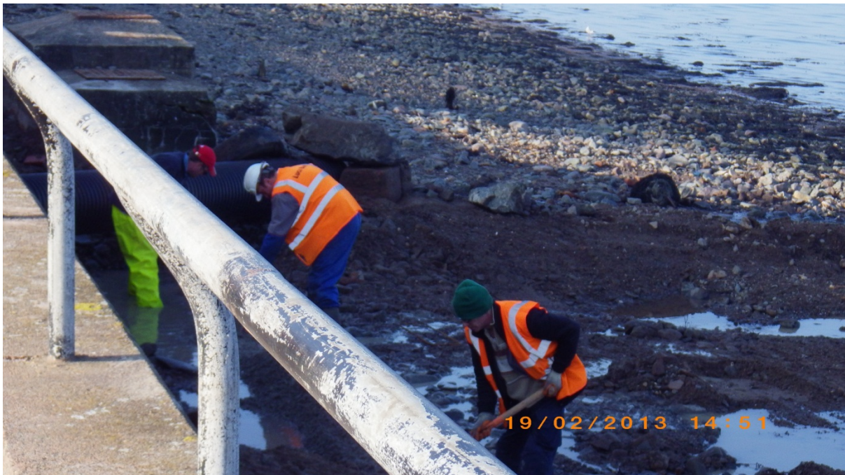
Figure 13. Storm drain replacement work. Waypoint 22.
