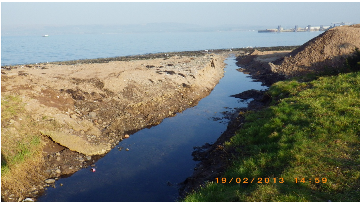
Figure 16. Discharge from large pipe. Waypoint 25.
