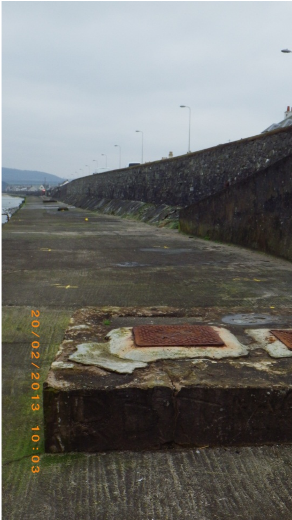
Figure 22. Manhole covers in seawall in Stranraer. Waypoint 33.
