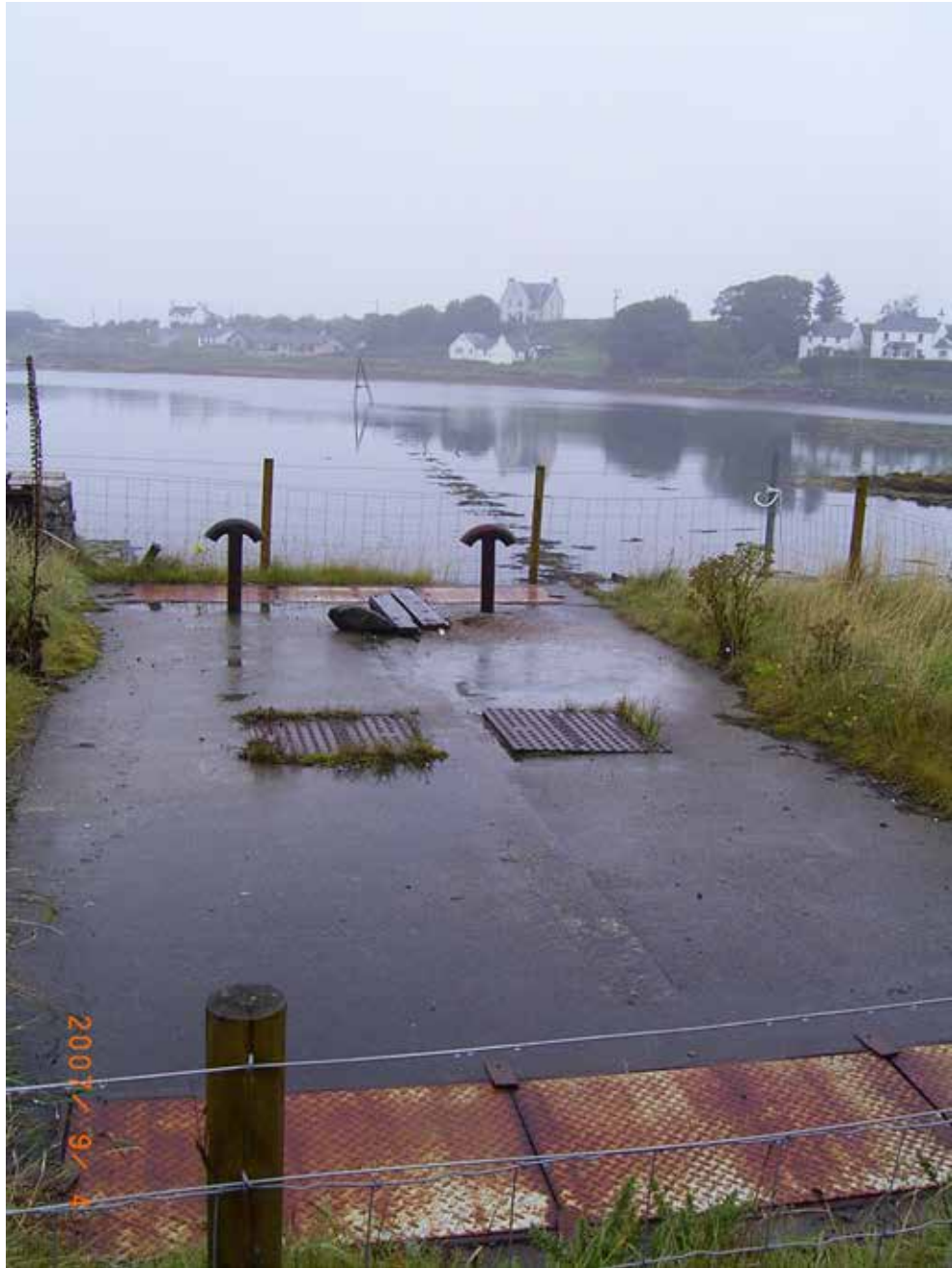
Figure 9. Bunessan communal septic tank
