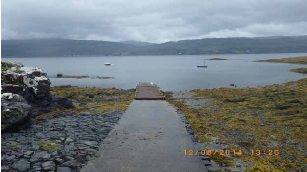
Figure 8: Pier below Killiemore House, WP 29.
