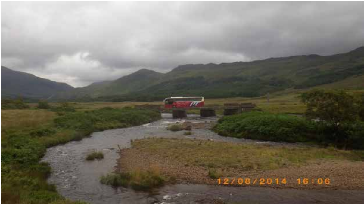
Figure 14: Modern road bridge carrying A849 road over the Coladoir River. Site of LSF07 (WP 58).
