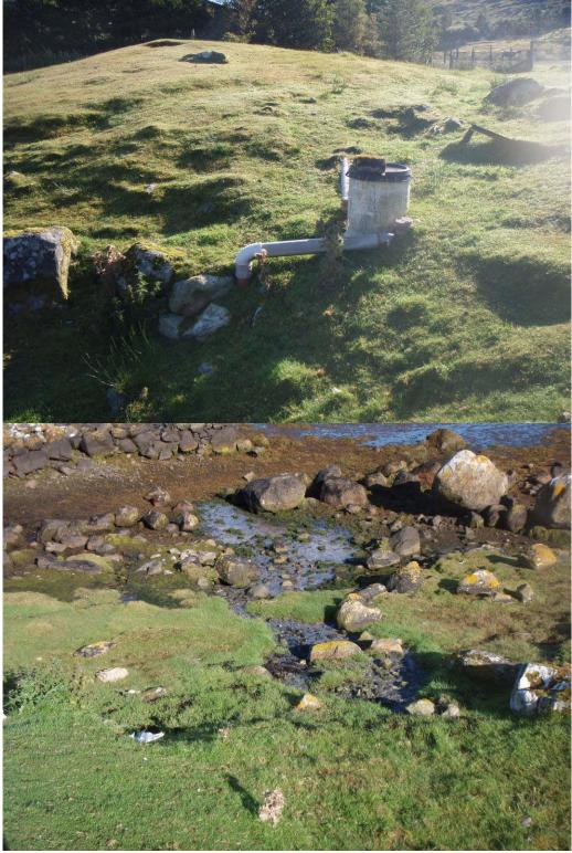
Figure 6. Septic tank head and leak at base
