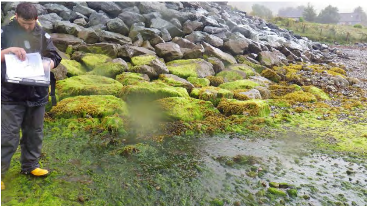
Figure 10. Water flow from below septic tank at car park, Sconser Pier. Site of LSF5. Associated with WP22.
