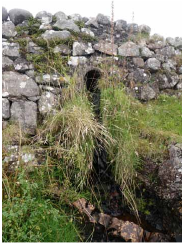
Figure 7. Culvert through road
