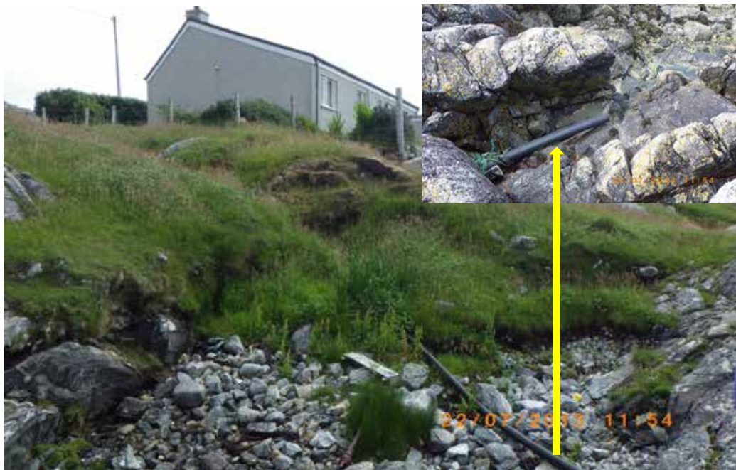
Figures 6&7. Sewage pipe from dwelling (insert), pipe outflow onto shore. Waypoint 8.
