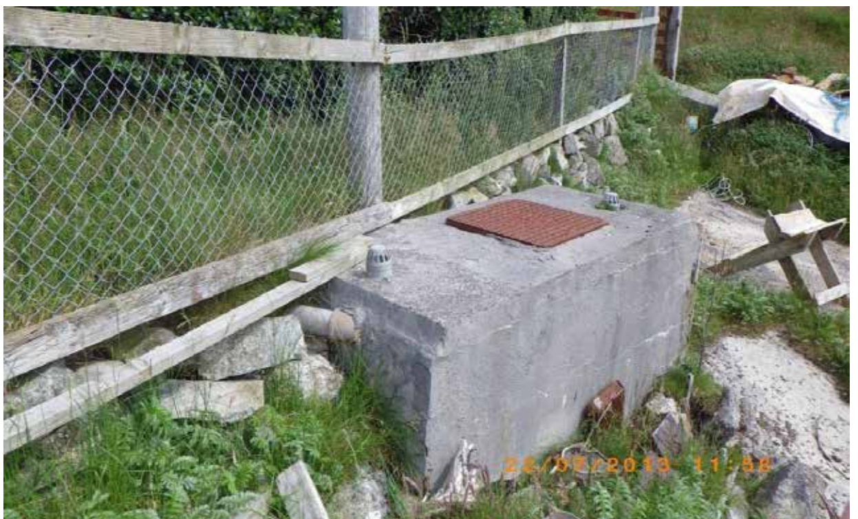
Figure 9. Septic tank also from same dwelling as Figures 6, 7 & 8. Waypoint 10.
