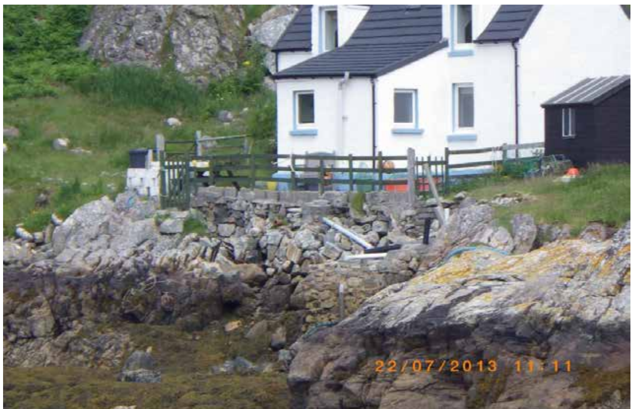
Figure 4. Sewage pipe from house to harbour. Waypoint 4.
