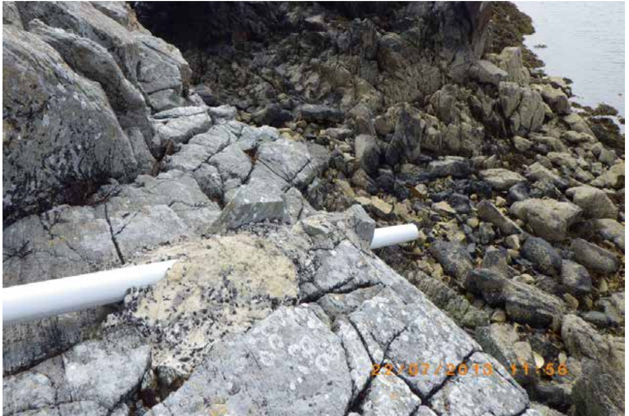
Figure 8. Another pipe from same dwelling in Fig 6 & 7, no outflow. Waypoint 9.
