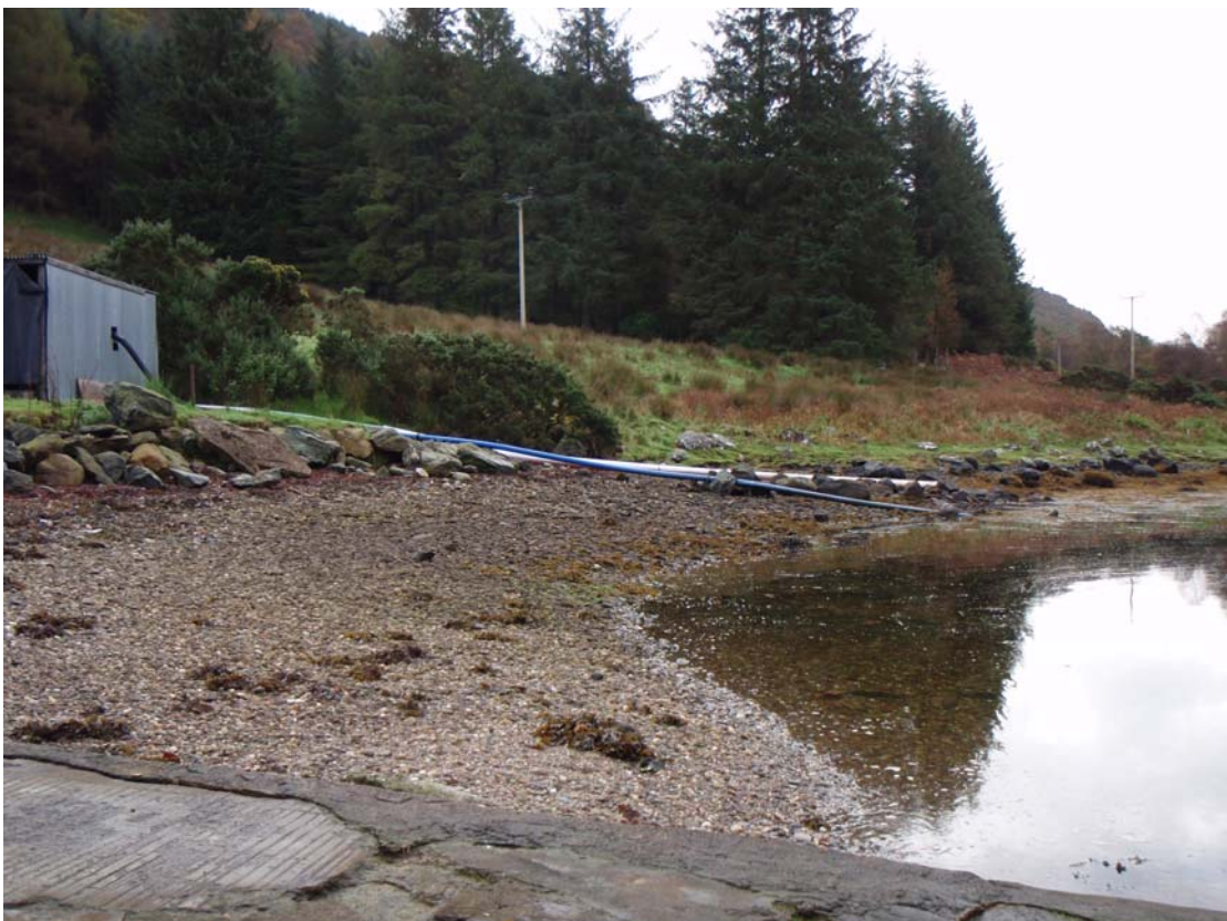
Figure 7. Slipway and disused deputation shed
