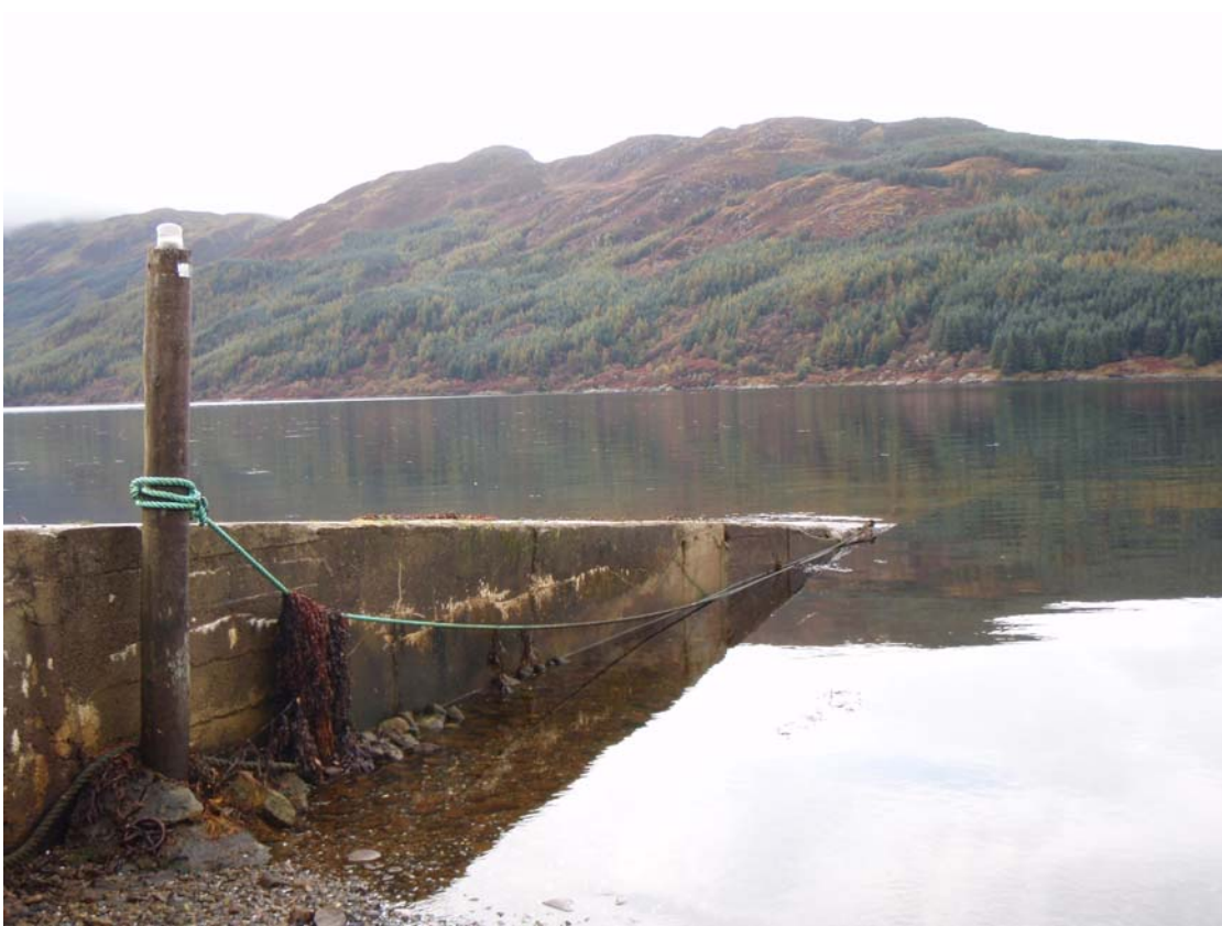
Figure 29. Slipway at Ardtaraig
