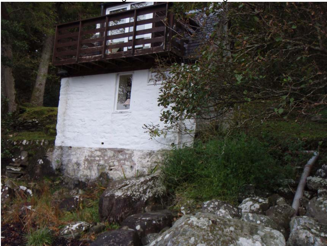
Figure 20. Small cottage with pipe leading to the shore
