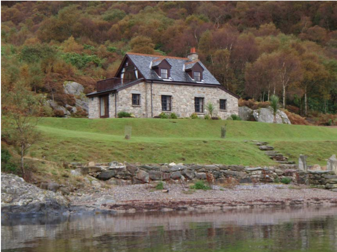
Figure 23. Large house with no apparent discharge pipes
