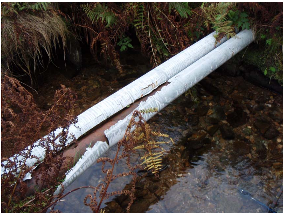
Figure 25. Stream with pipes running across it.
