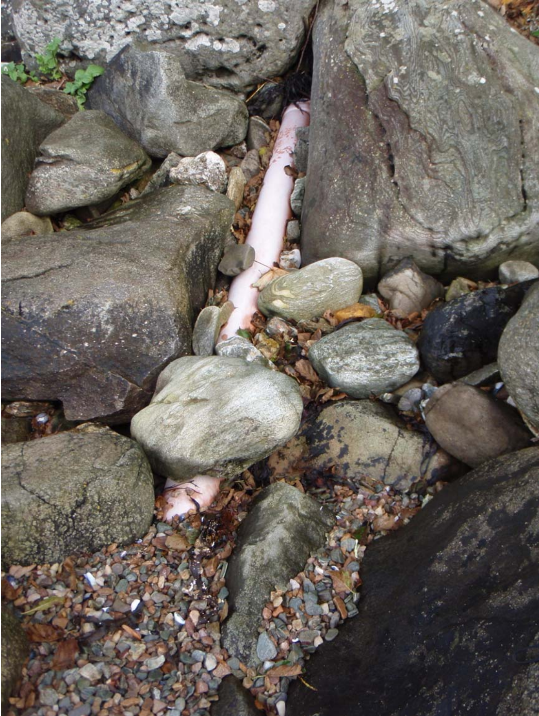
Figure 22. Discharge pipe across shore
