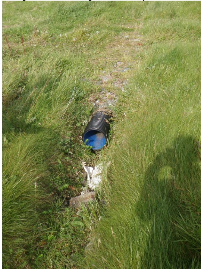
Figure 13 Culvert pipe above drainage ditch, dry at time of survey
