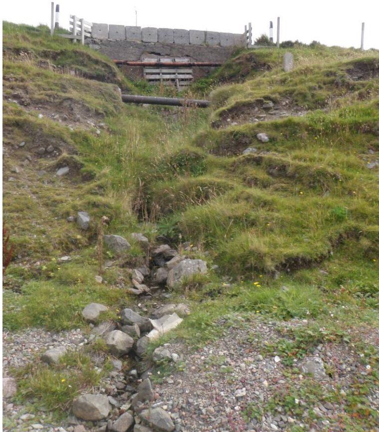
Figure 20 Dry stream bed under road
