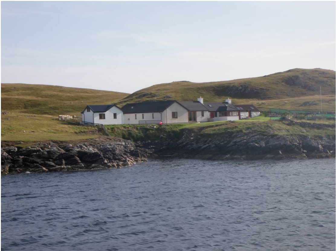
Figure 9 House and septic tank
