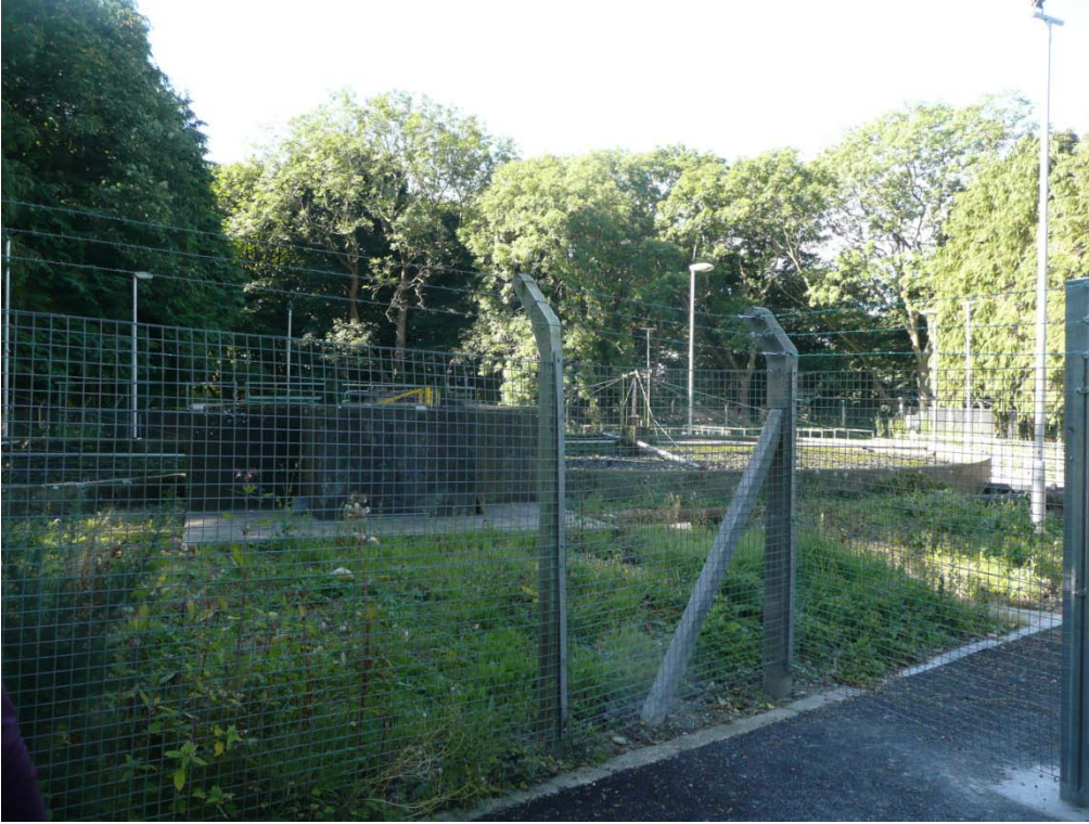
Figure 18. Glenluce sewage works
