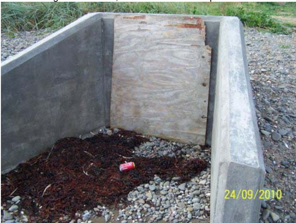
Figure 9. New culvert – boarded up
