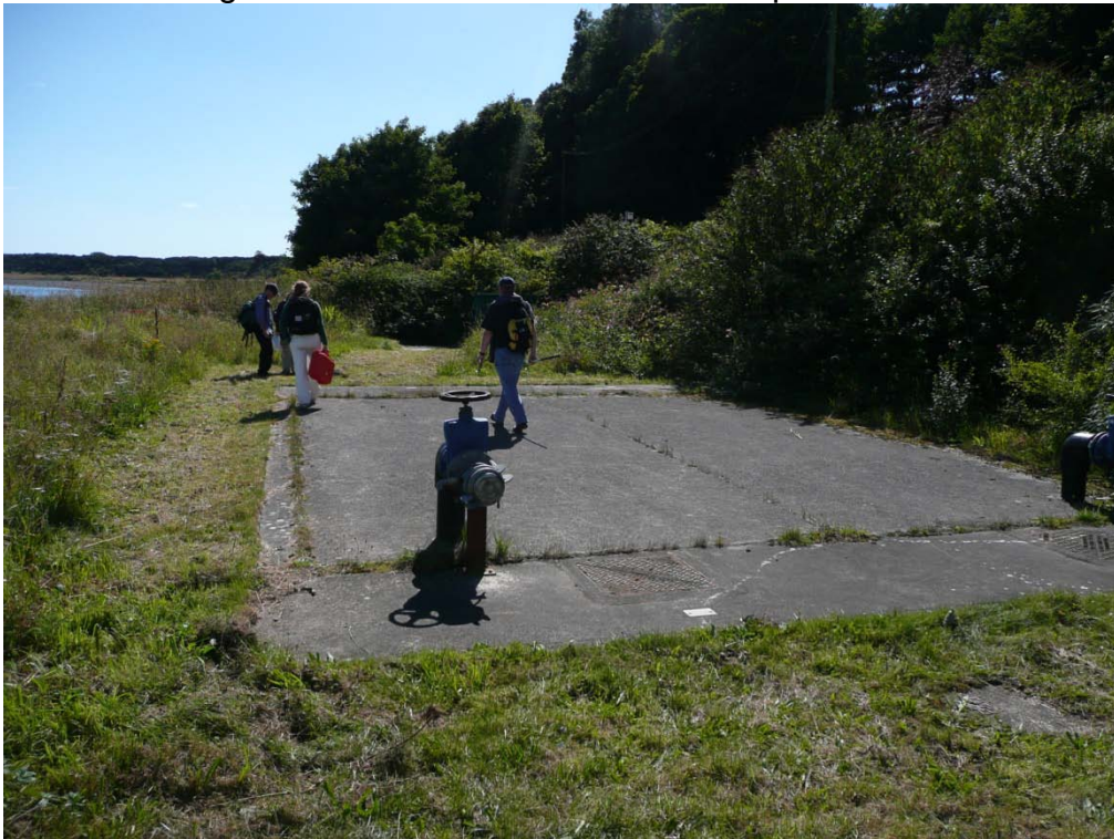
Figure 11. Sandhead septic tank
