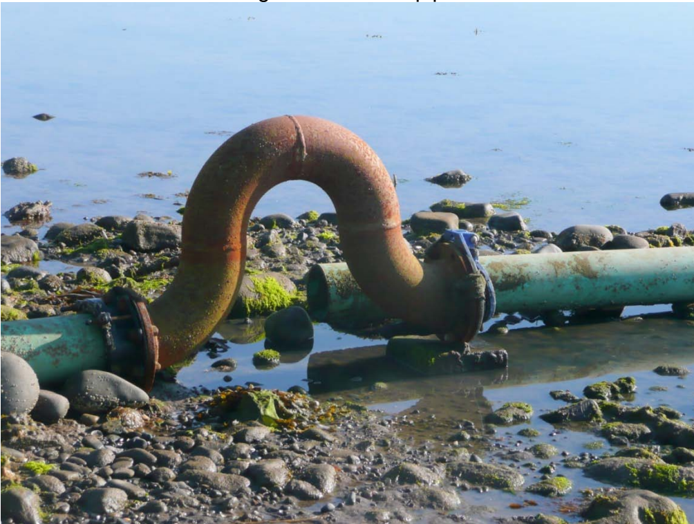
Figure 15. Link in outfall pipe, shown in Figure 14
