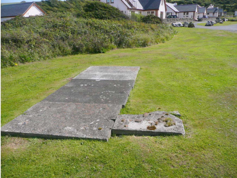
Figure 20. Stairhaven septic tank
