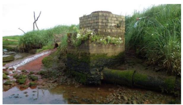
Figure 17 Inspection junction in pipe (leaking) connecting with St. Andrews Caravan Park PS EO. Location of unplanned freshwater sample MCFW8, Waypoint 39.
