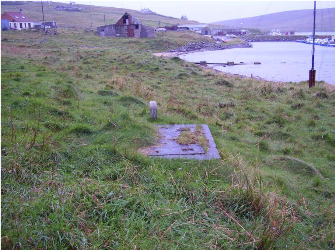
Figure 16. Tank cover. discharge pipe, and marina.
