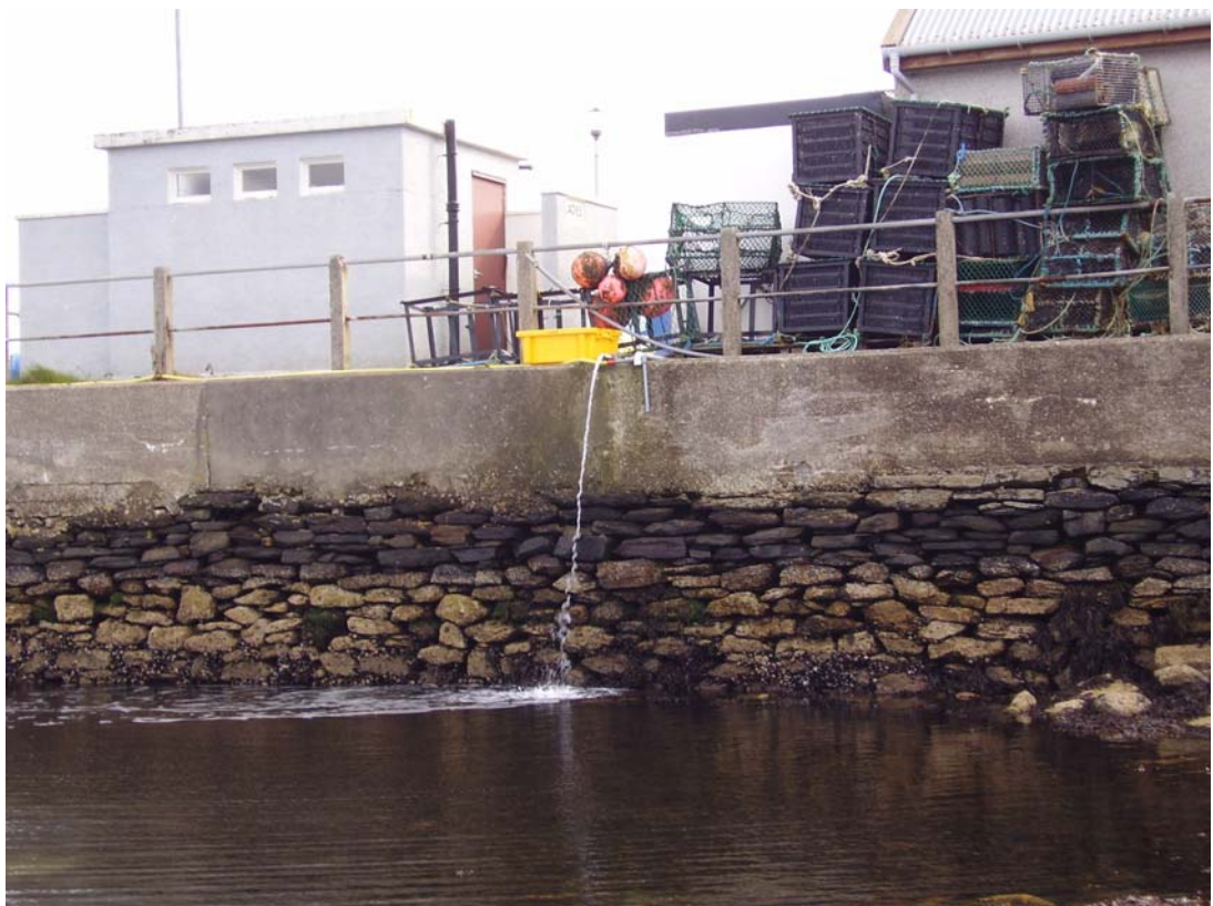
Figure 13. Discharge at pier.
