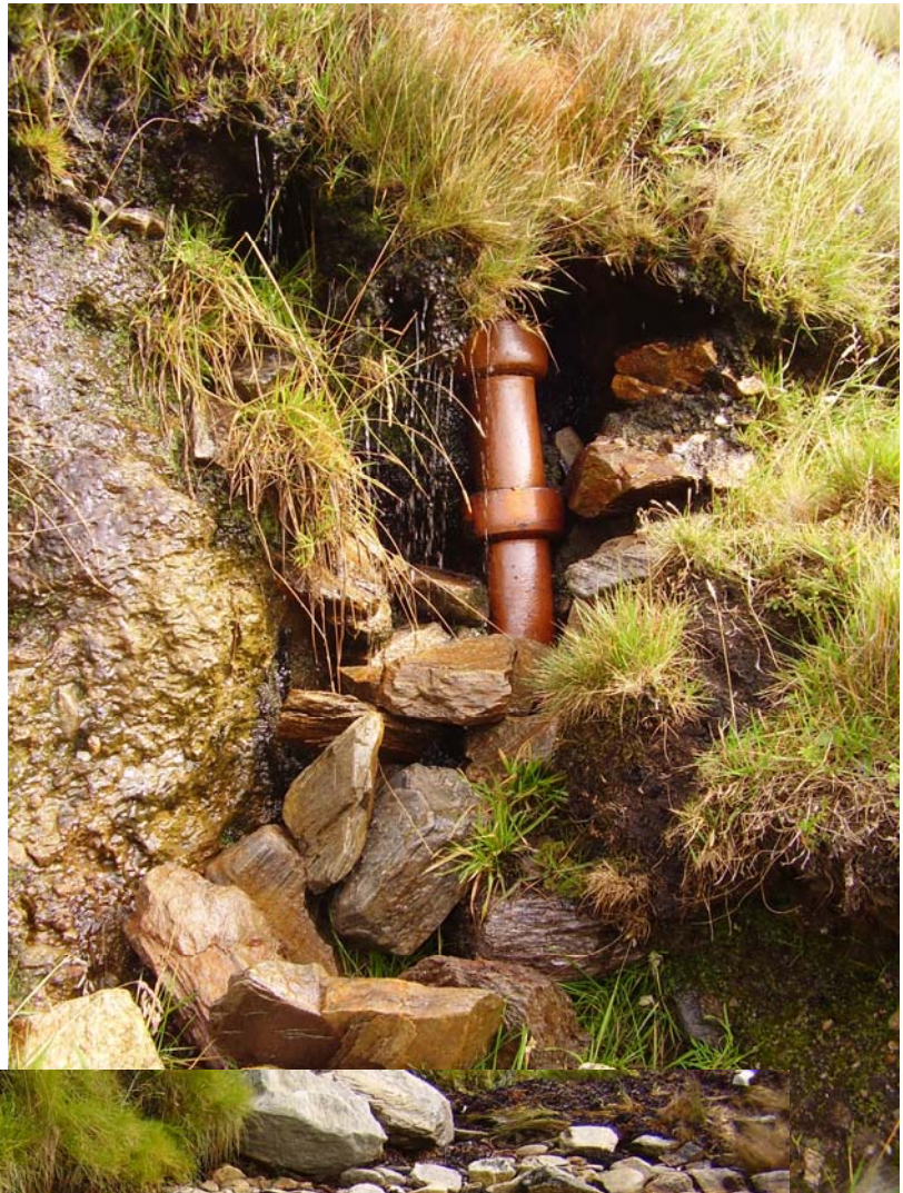
Figure 24. Vertical section of pipe discharging onto shoreline
