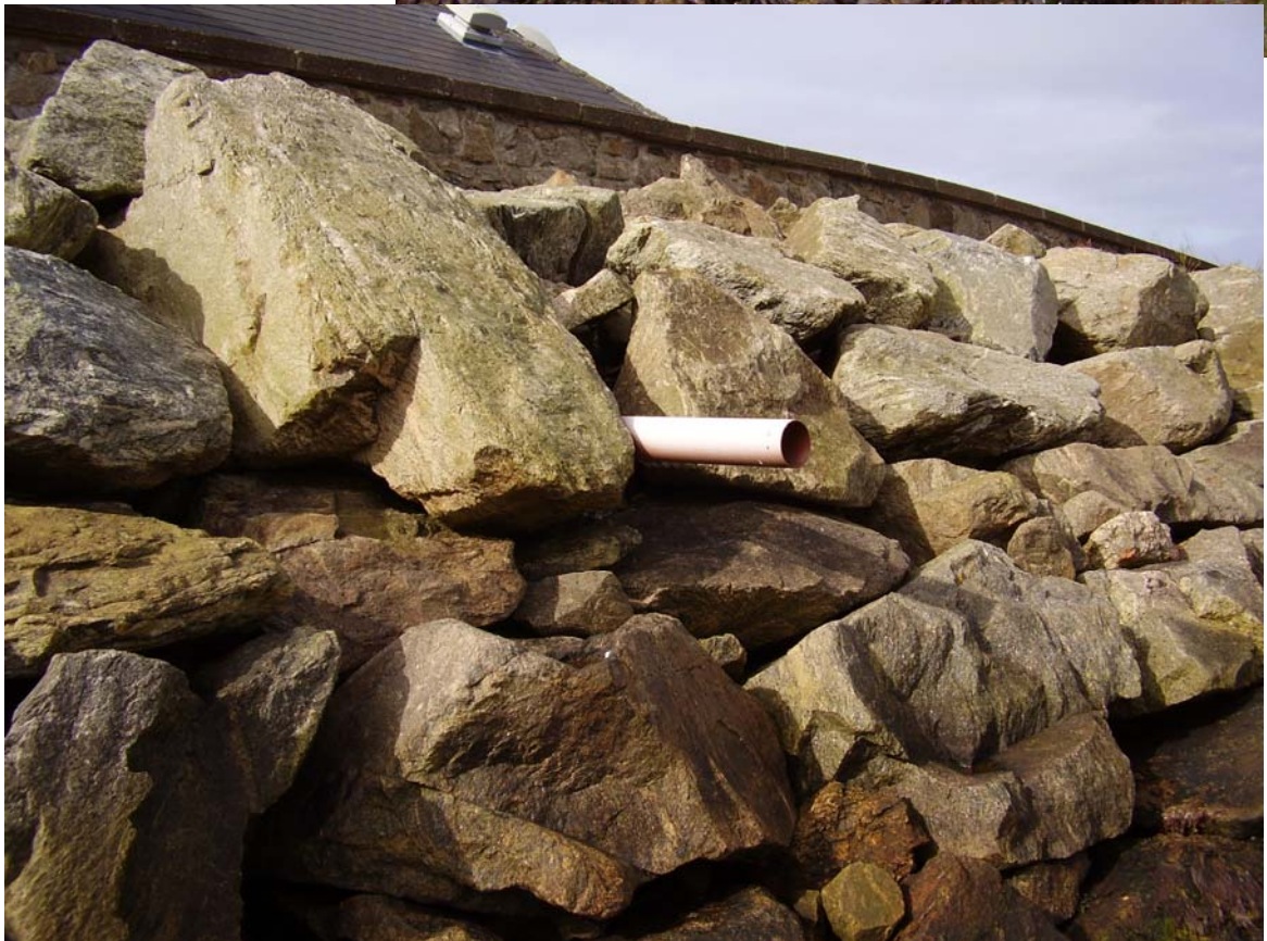
Figure 11. Drain pipe through seawall.
