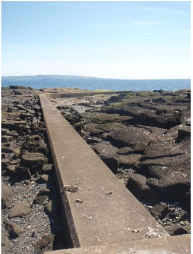
Figure 15. Scottish Water discharge outfall pipe, with spat growing in end of pipe, location of sea water sample NBSW4
