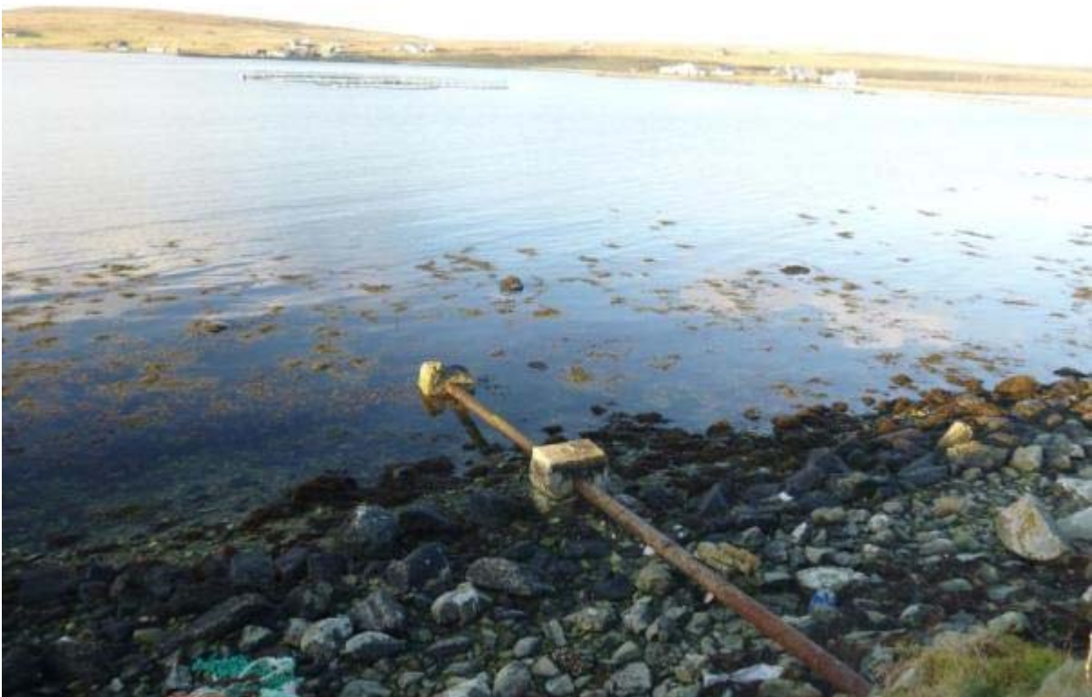
Figure 11 – Outlet pipe below 1 dwelling house on eastern coastline (no discharge).
