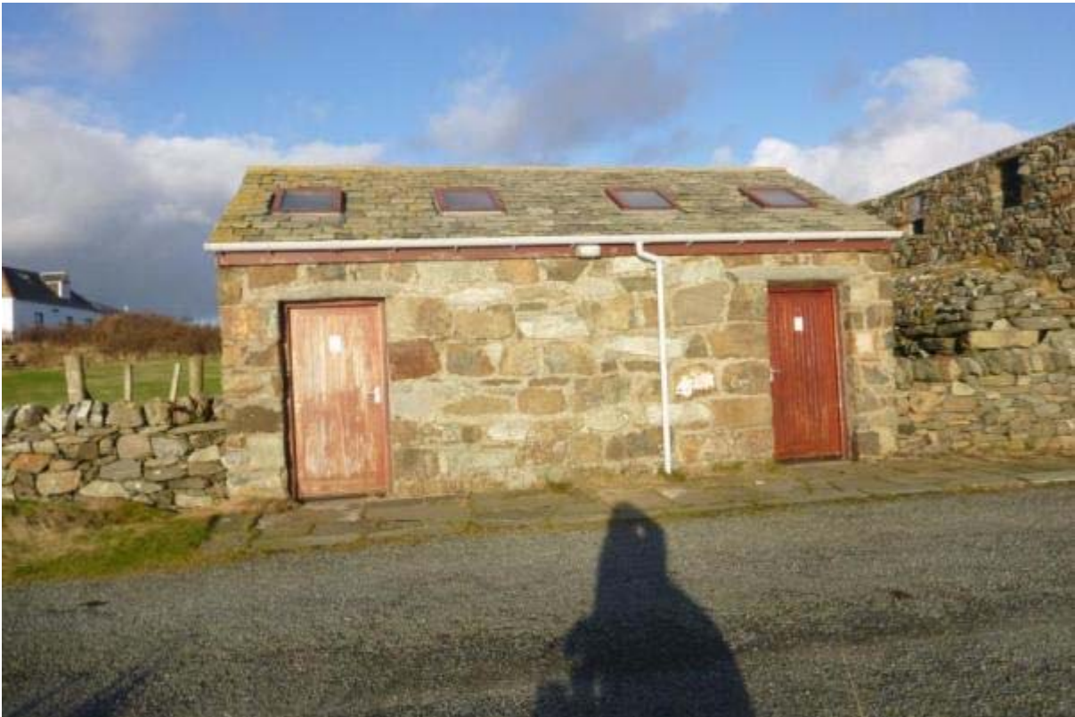
Figure 14 – Public toilets beyond the Westside pier.
