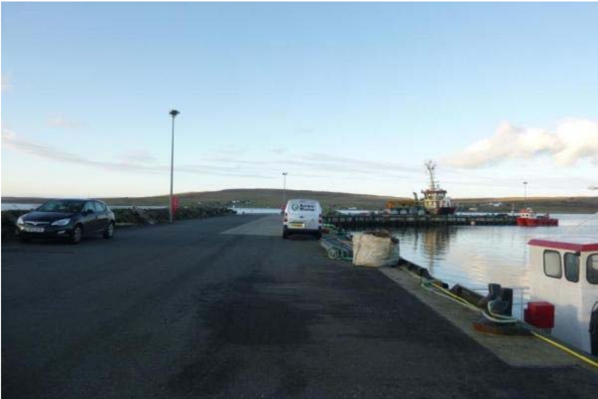
Figure 22 – Workboats at Uyeasound Pier.
