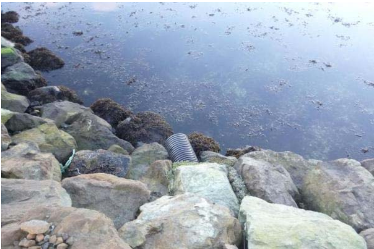
Figure 9 – Plastic pipe (no outflow) near Uyeasound Pier.
