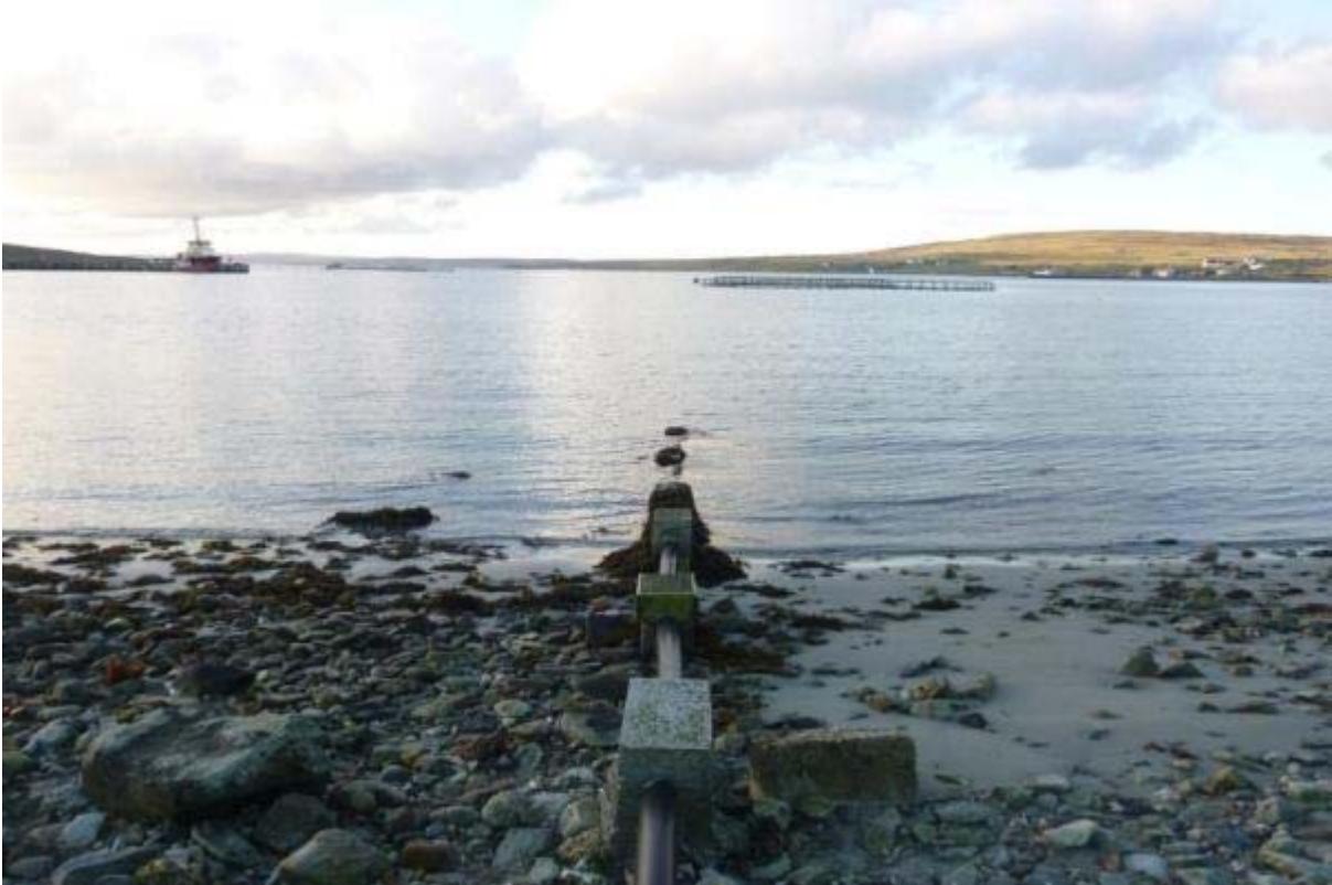
Figure 12 – Possible sewage pipe to the east of Easter Loch.
