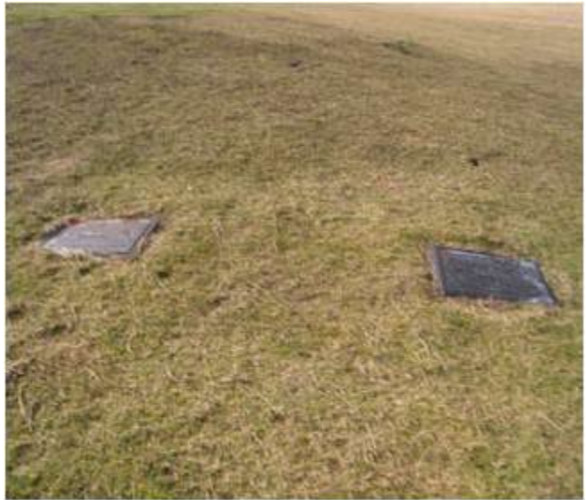
Figure 10. NG 01960 93790 looking NW Figure 11. Inspection covers for septic tank at golf course
