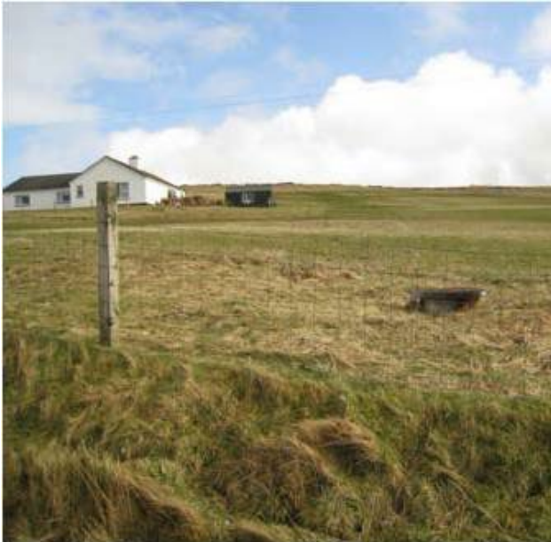
Figure 14. Septic tank at NG 01140 93270
