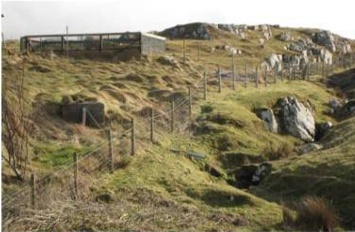
Figure 4. Septic tank at NG 02670 94080
