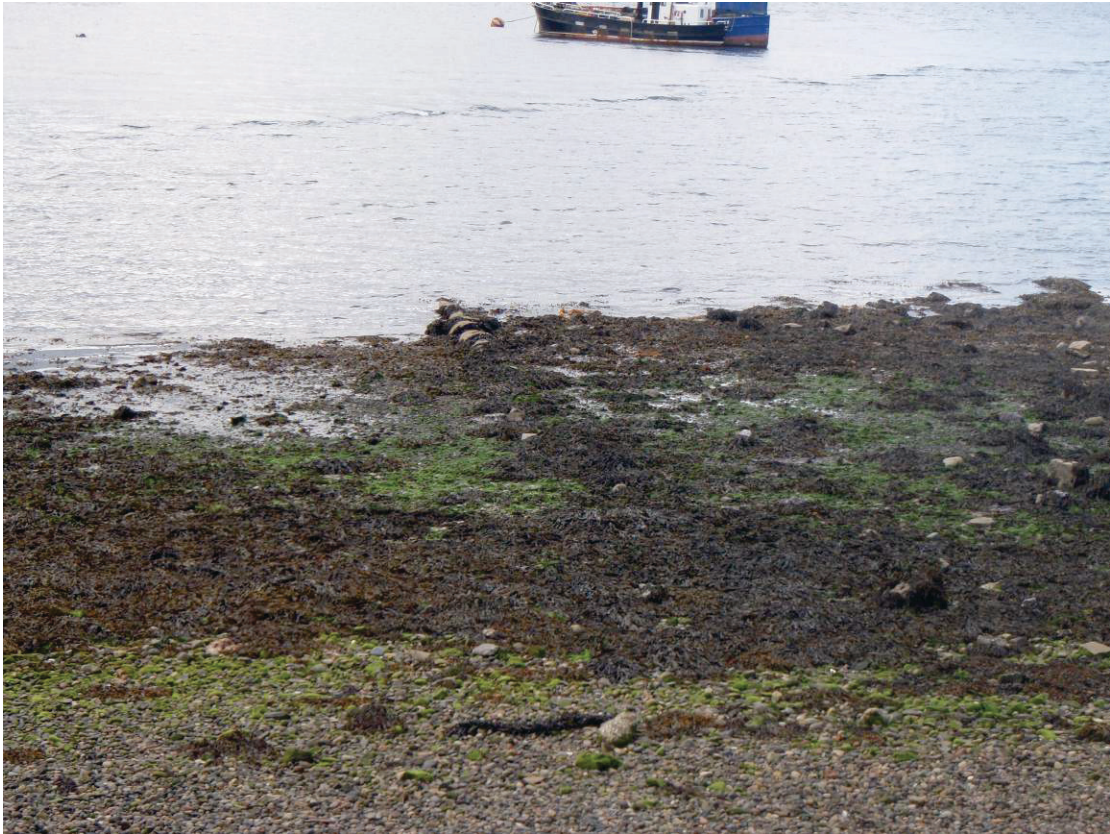
Figure 24. Pipe running across beach which appeared redundant
