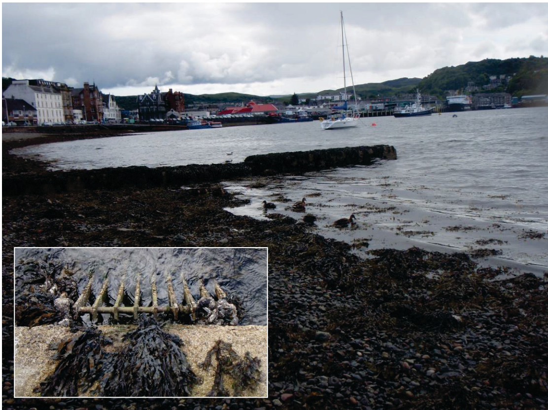
Figure 25. Possible outfall pipe running across beach with grill at the end (inset)
