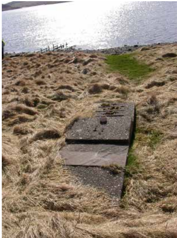
Figure 12 – Septic tank below an occupied property at Olna.
