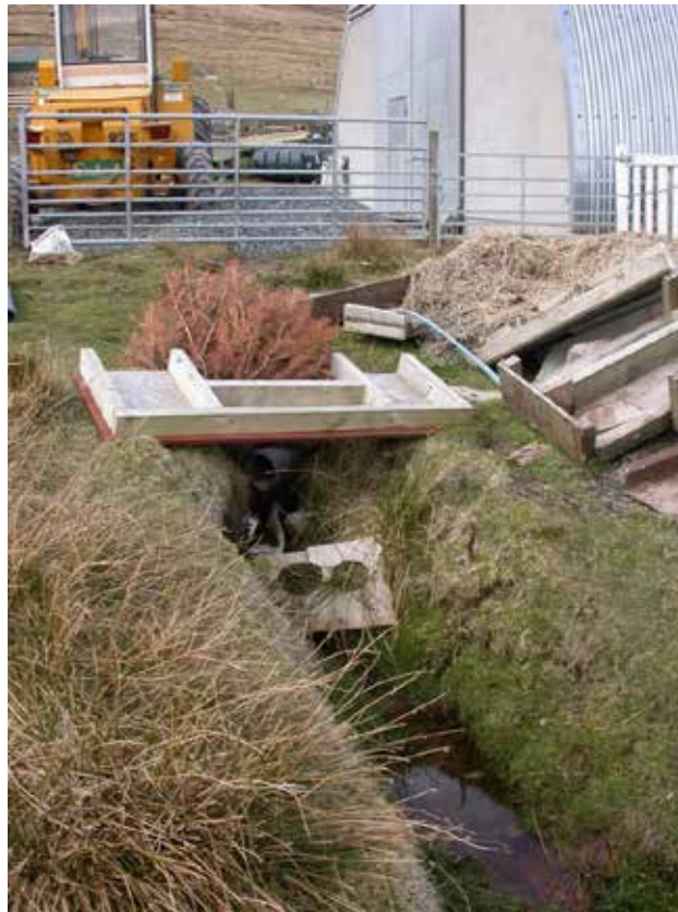
Figure 14 – Drain leading to the shore from an agricultural building at Hoga.
