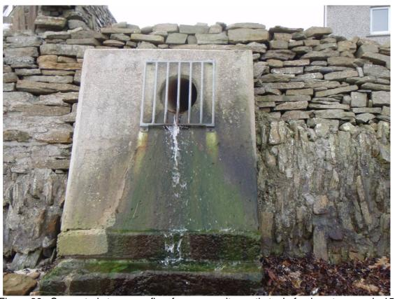
Figure 30. Suspected storm overflow for community septic tank, fresh water sample 15
