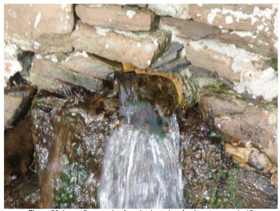
Figure 26. Large flow coming from broken pipe, fresh water sample 12
