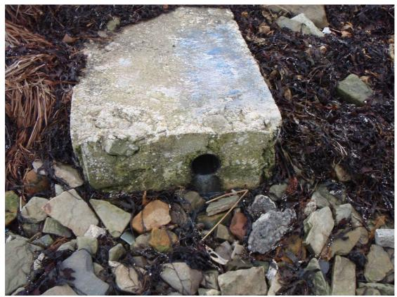
Figure 35. Pipe encased in concrete, sewage fungus, fresh water sample 18
