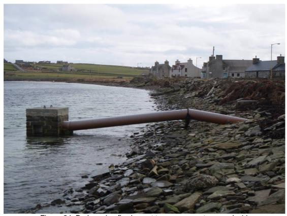
Figure 34. Broken pipe flowing out to sea, sea water sample 11
