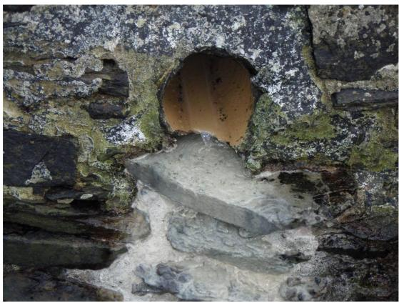
Figure 39. Broken pipe with sewage fungus, fresh water sample 21
