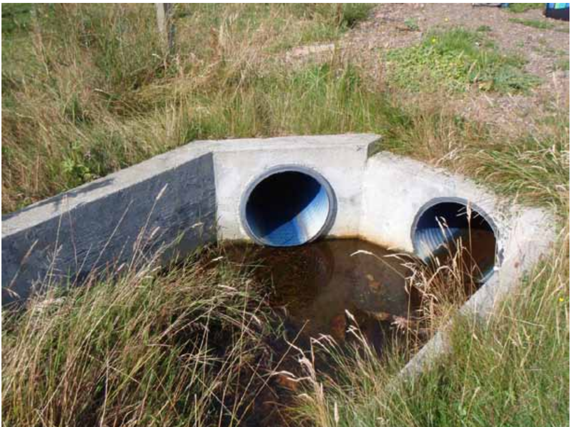
Figure 19. Two culverts running into stream shown in Figure 17
