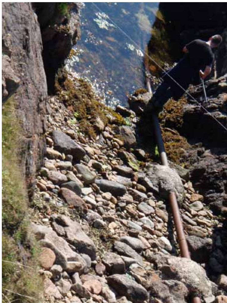
Figure 9. Iron pipe flowing into the sea, location of seawater sample MRSW3
