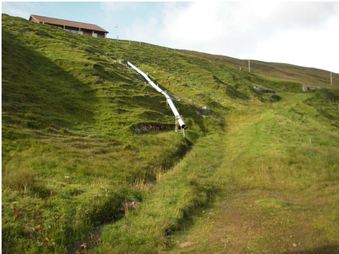
Figure 17. Ronas Voe-0064. Pipe below dwelling
