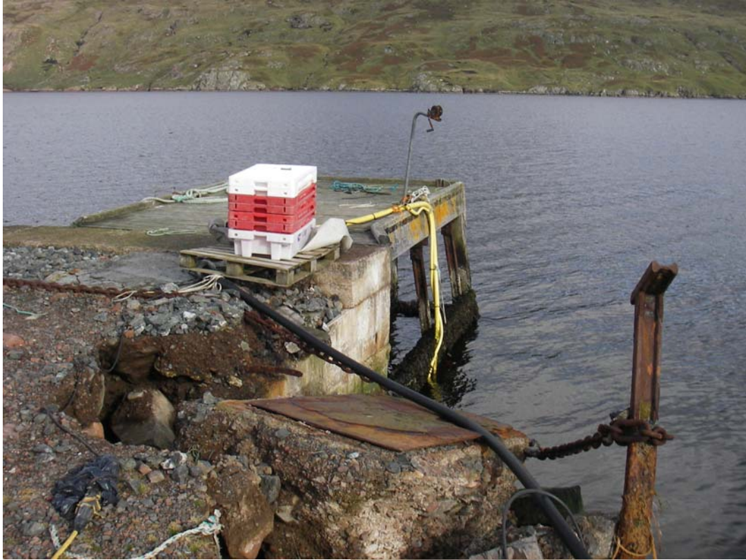
Figure 15. Ronas Voe-0061 Pipe below Aquafarms Ltd.
