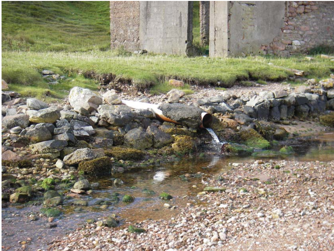
Figure 16. Ronas Voe-0063. Stream and pipe
