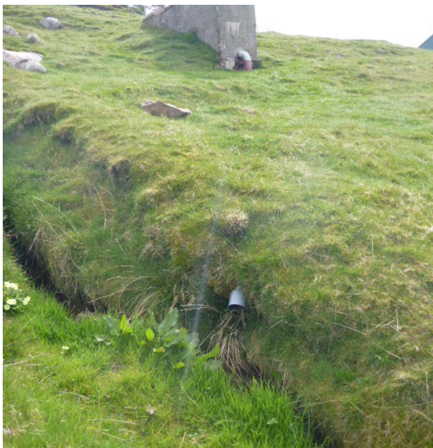
Figure 9 – Pipe assumed to be associated with a septic tank entering a small watercourse leading to the shore at the south end of Sandsound Voe.
