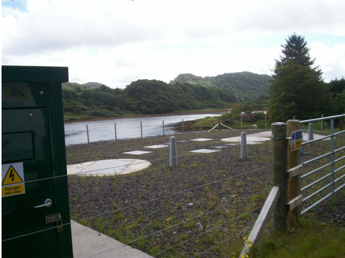
Figure 16. Clachan seil sewage works
